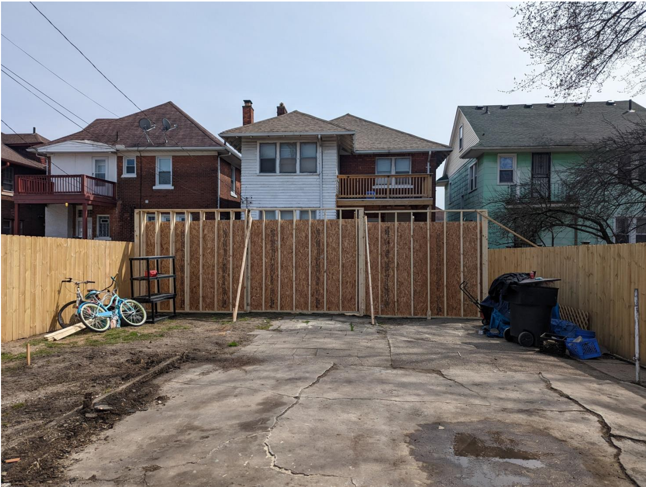
Figure 15 - Completed Demolition - Temporary Fence to limit access for property
