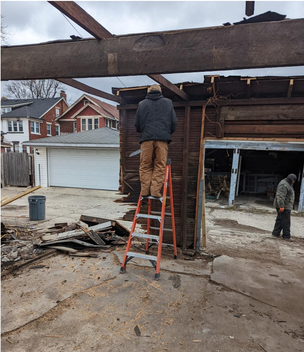
Figure 11 - Nearing demolition completion
