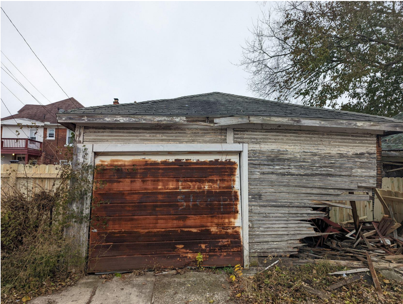
Figure 3 - Back of Garage (alley side) - see corner
