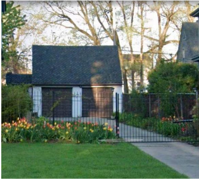
Garage, front elevation, facing Seminole, applicant photo
