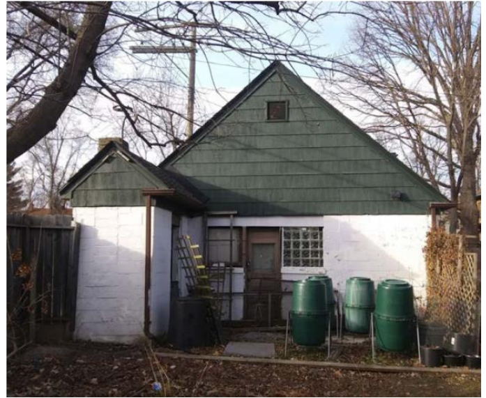
Garage, south elevation, applicant photo
