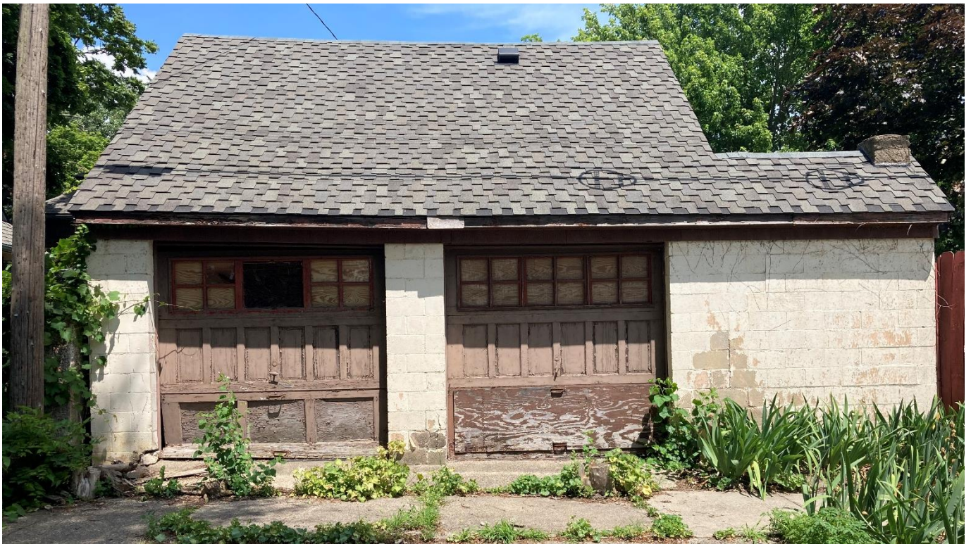
2151 Seminole garage, rear elevation (facing Maxwell), 7/2/2022 staff photo
