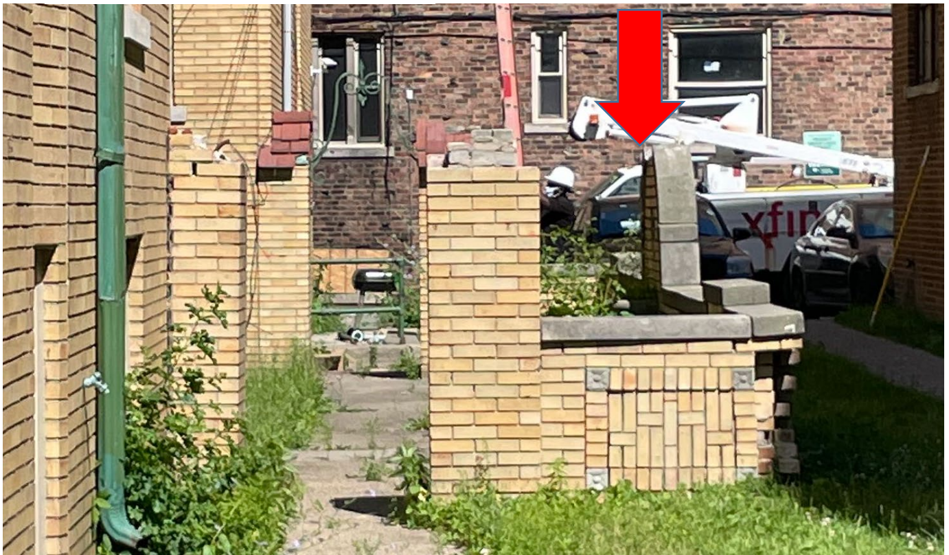
Site Photo 3, by Staff June 24, 2022: (South) Rear elevation, showing current conditions of the courtyard and wall fountain (red arrow), visible from the public sidewalk on Third Street.
