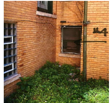
Site photo 7, by Applicant, (rear, west-facing elevation), showing proposed location for window replacement with glass block, #4.
