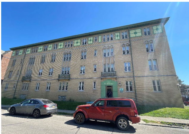
Site Photo 1, by Staff June 24, 2022: (North) Front elevation, showing original casement windows.
