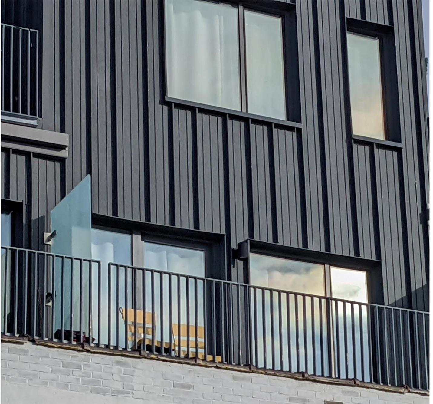
**Example of Kalzip standing seam product in situ at 644 Selden. The Commission approved this siding for installation at 655 W. Willis at the 4/10/2019 meeting. Note the pronounced shadow lines which result from the height of the standing seam and pencil ribs**
