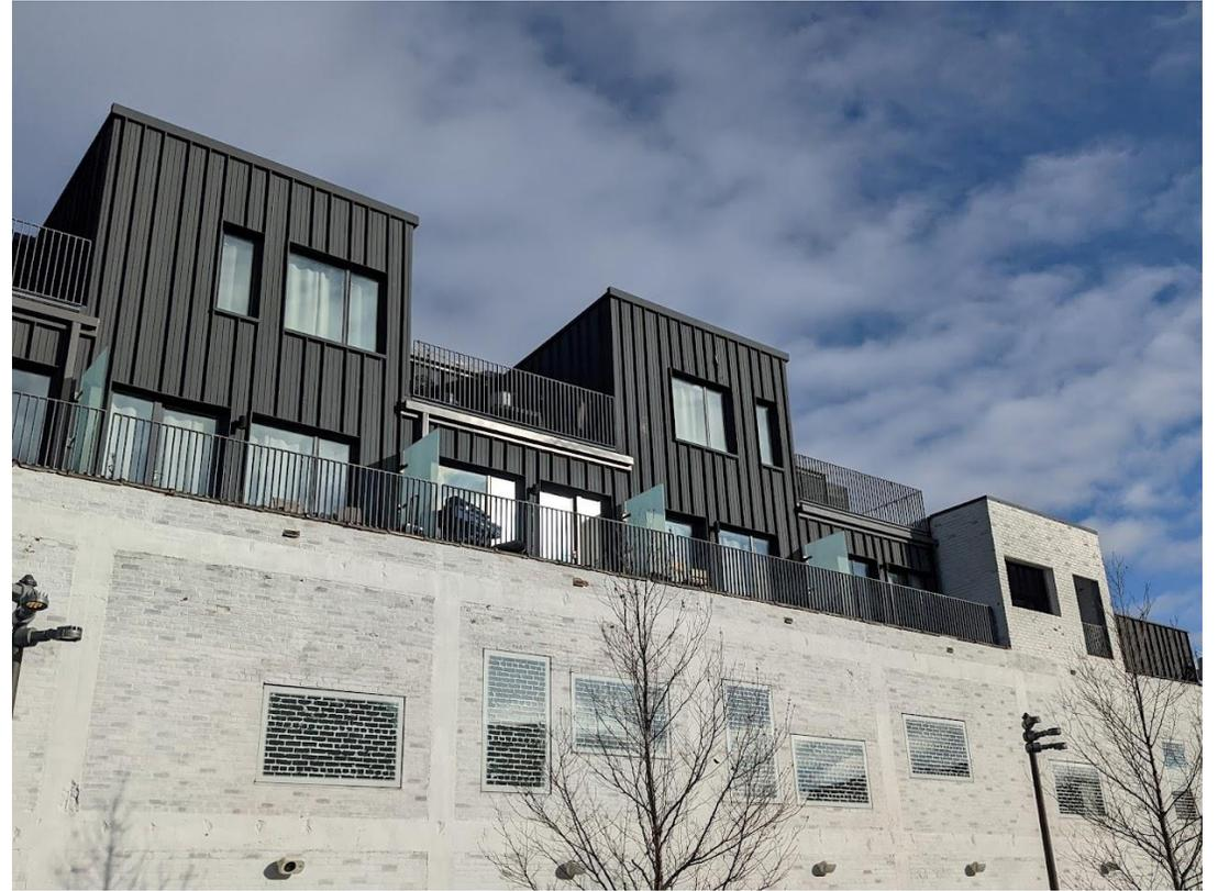
**Example of Kalzip standing seam product in situ at 644 Selden. The Commission approved this siding for installation at 655 W. Willis at the 4/10/2019 meeting. Note the pronounced shadow lines which result from the height of the standing seam and pencil ribs**
