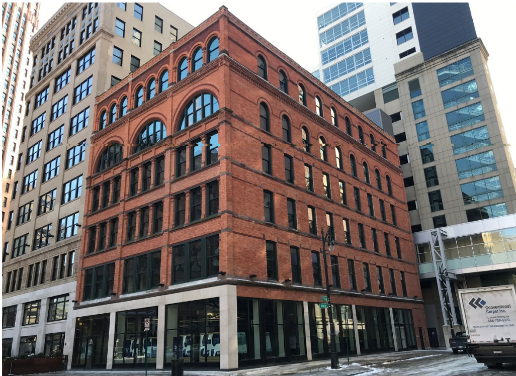
View of existing conditions at 119 State, corner of Shelby Street and State Street. Staff photo, February 15, 2022.
