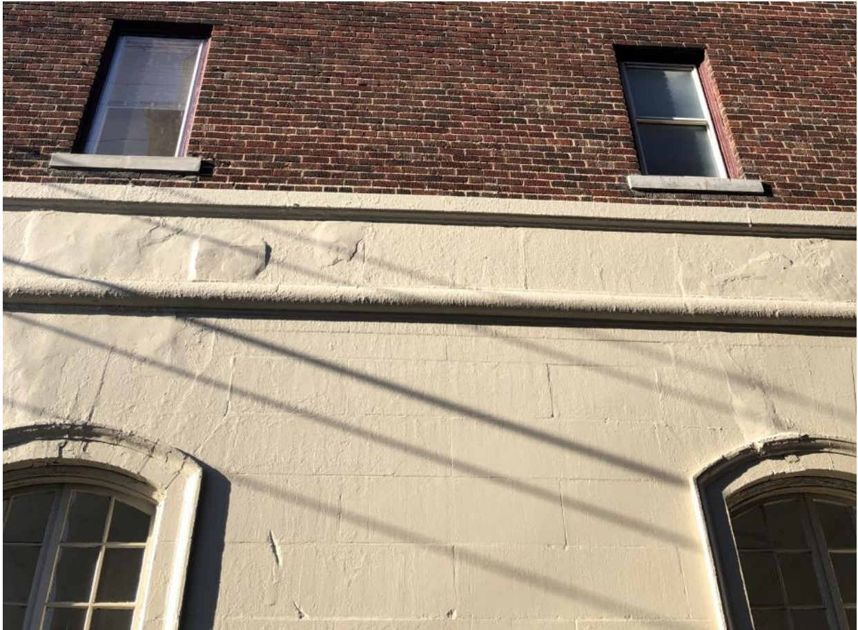
In this January 2022 HDC staff photo, poor repair/patching work was completed and then covered with a coating that minimizes the stone block pattern (which is now only noticeable up close), and obliterates the contrasting beveled stone detail above the arched window. This surface treatment was in place at time of district designation.
