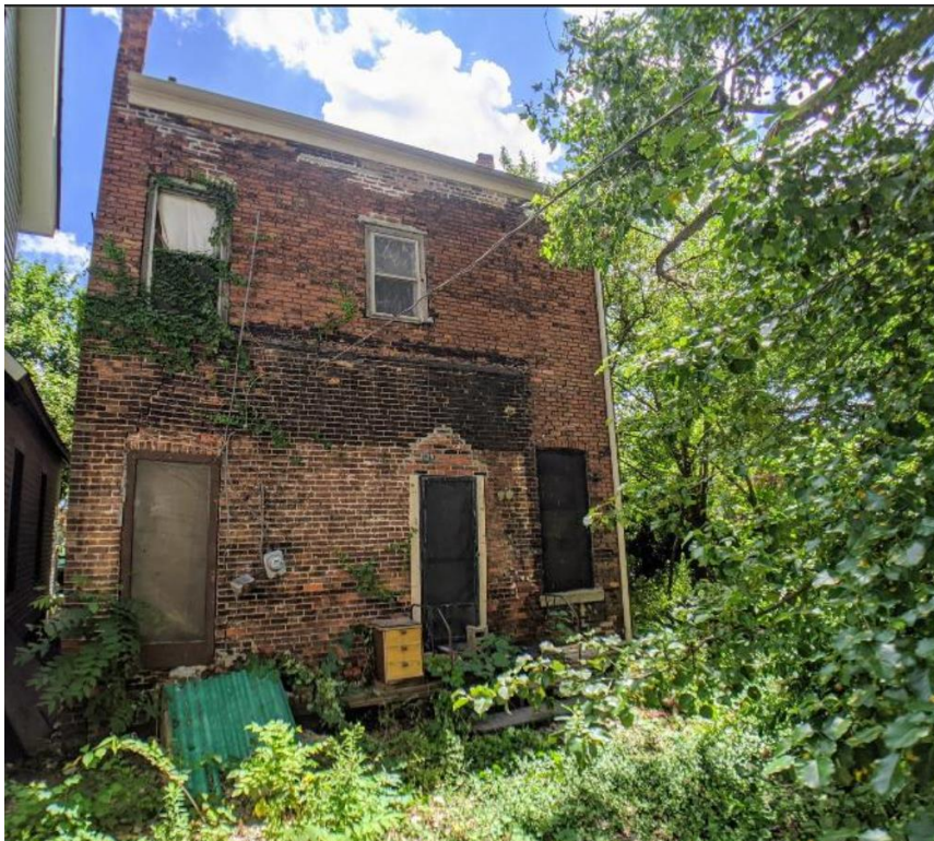
1356 Labrosse, appearance in 2020 prior to current brickwork
