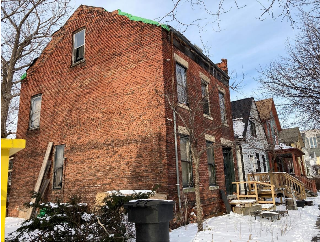
1356 Labrosse, current appearance (side/west elevation)
