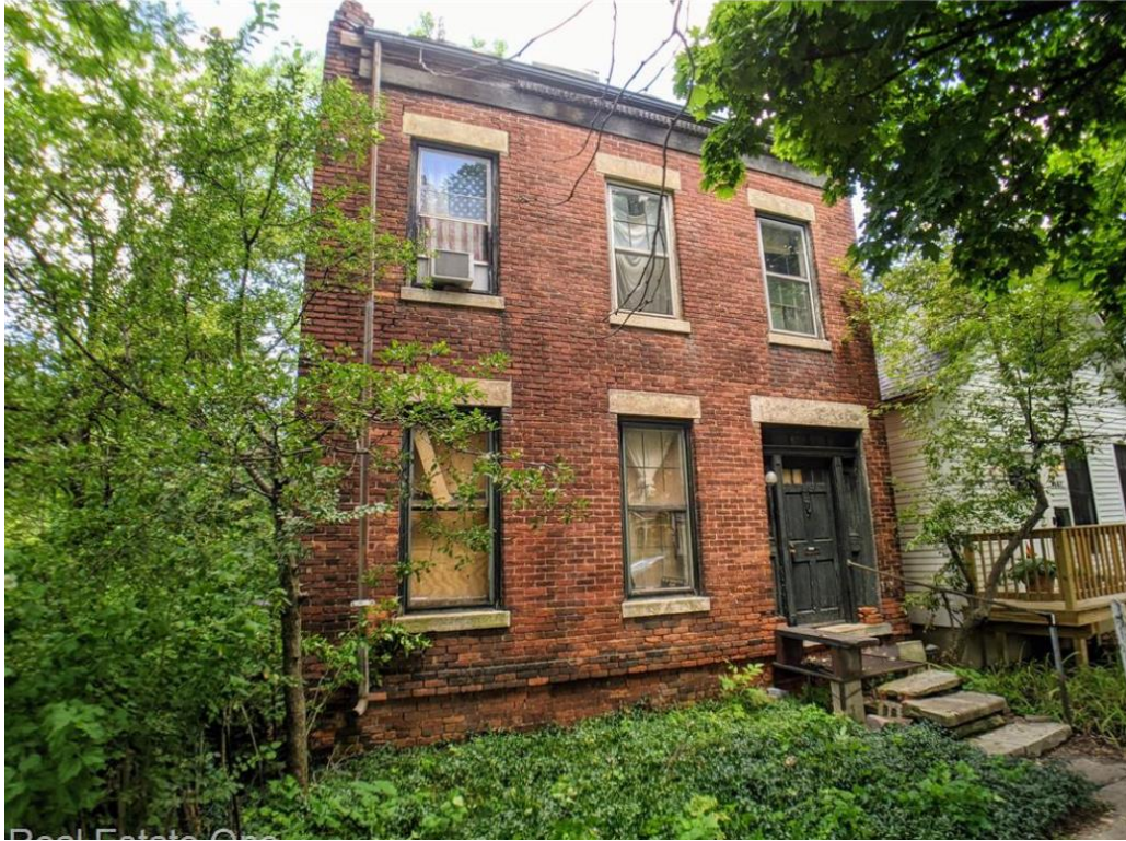
1356 Labrosse, appearance in 2020 prior to current brickwork
