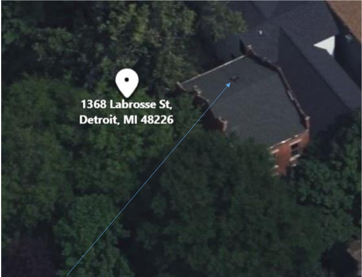
1368 Labrosse, showing existing rooftop skylight
