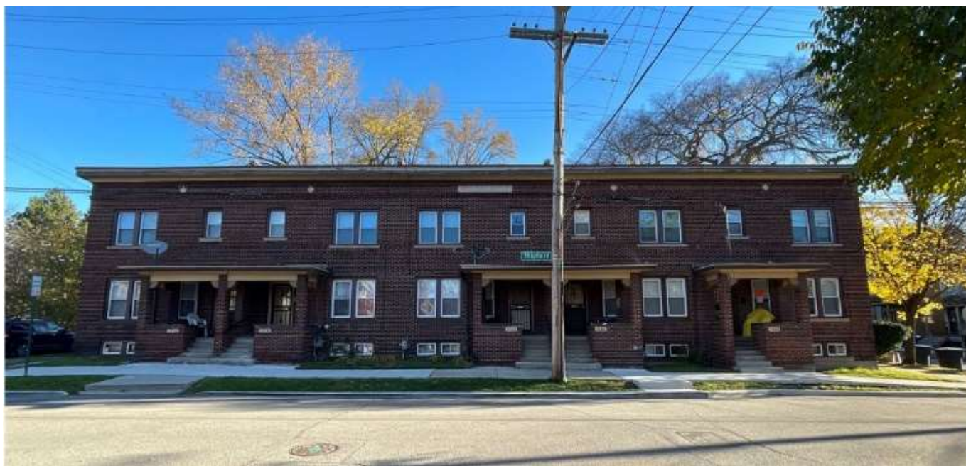
Site Photo 1, by Staff November 19, 2021: (Southwest) front elevation showing work complete of vinyl window installation and painted masonry on first floor window sills and capstones of the front porches. The BSEED stop work notice can be seen on the right-most entrance.
