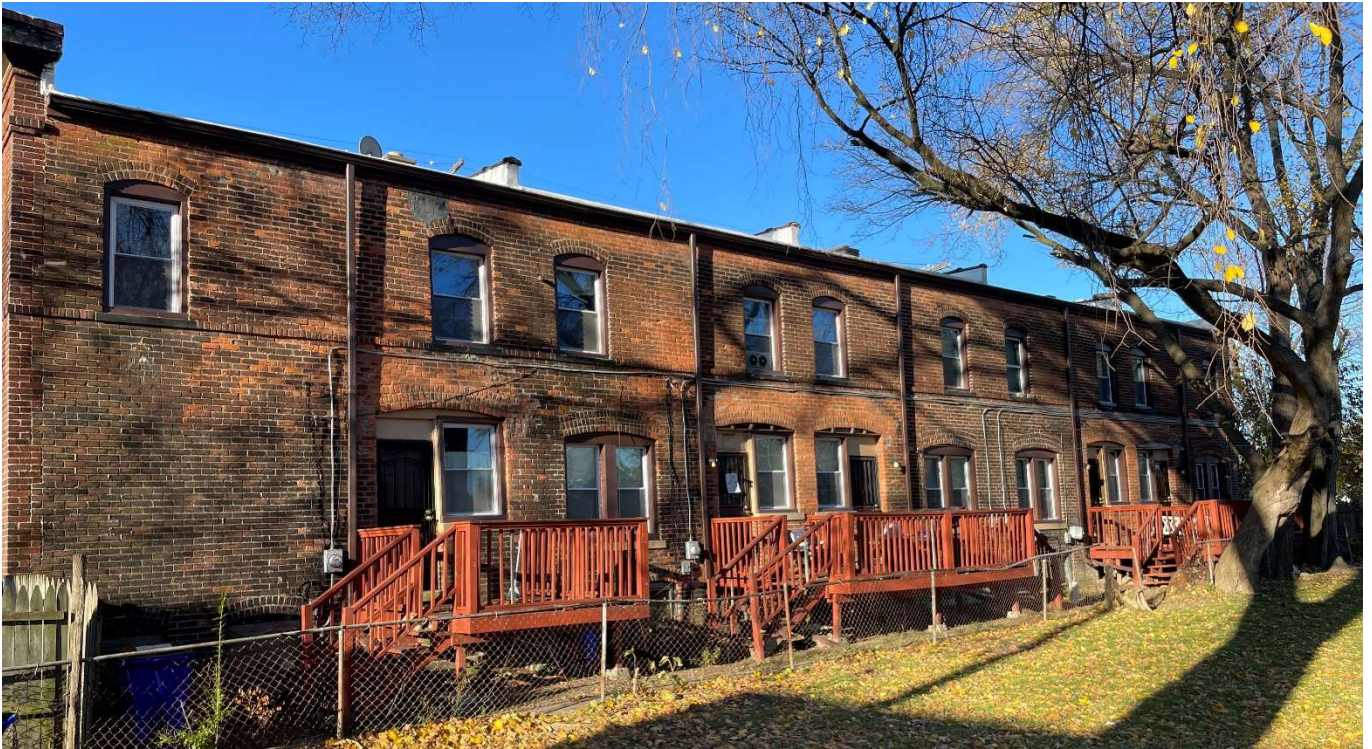
Site Photo 2, by Staff November 19, 2021: (Northeast) rear elevation showing installed vinyl windows on first and second floors.
