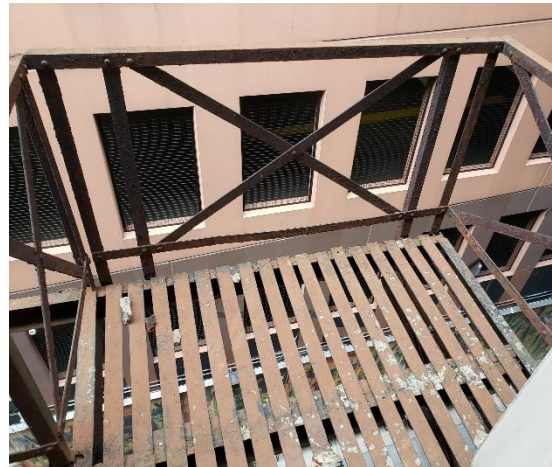
Figure 3: Rusted Rail
