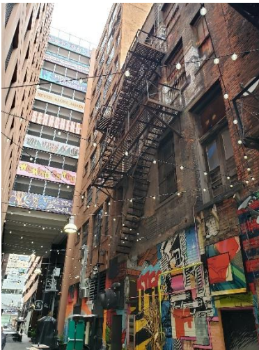
Figure 1: 1315 Broadway Fire Escape
