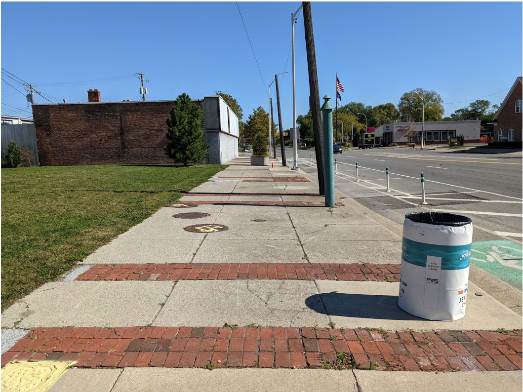
Current view in front of 14901 East Jefferson looking east towards Grosse Pointe Park. The brick sidewalk ornamentation was meant to enrich the pedestrian experience here and elsewhere in the district, but has lost the commercial street wall that previously framed it. Staff photo, October 1, 2021.
