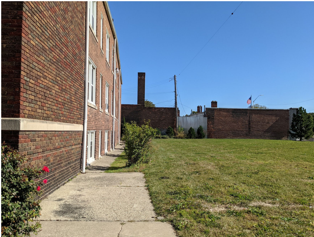
View to the east along south elevation of 1020 Alter, where loading drive is proposed. By staff's count, there are thirty-two (32) operable windows at this elevation, including several at grade. Staff Photo, October 1, 2021.
