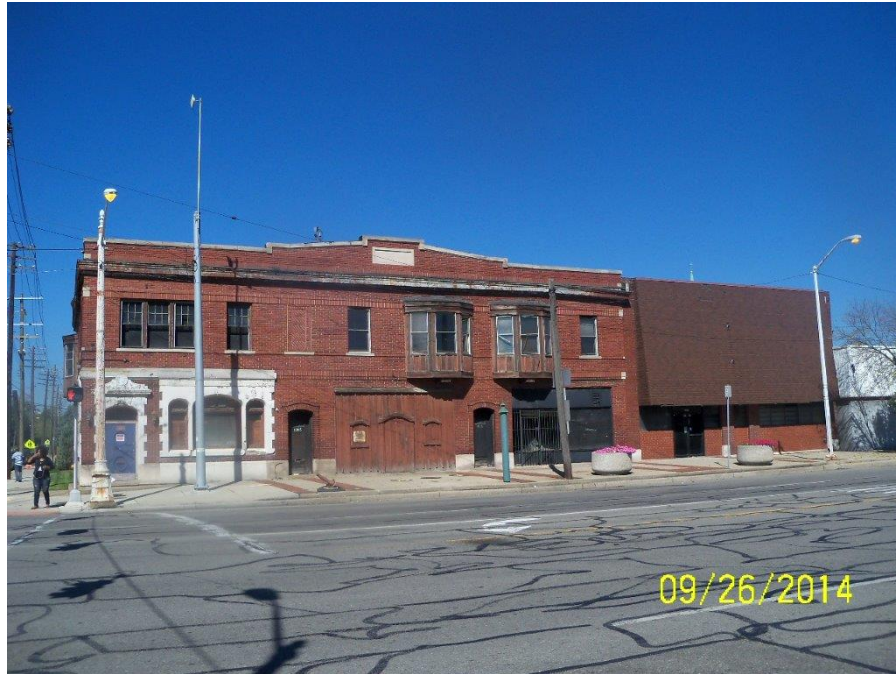
Photograph 3 – Exterior building façade off Jefferson Ave.
