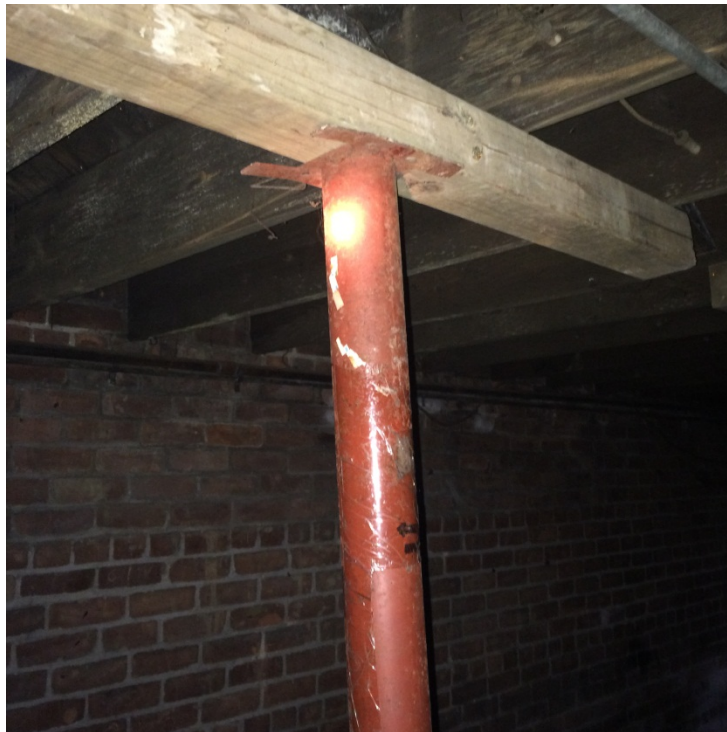
Photograph 12 – Basement – Additional jack post and wood framing under floor joists.
