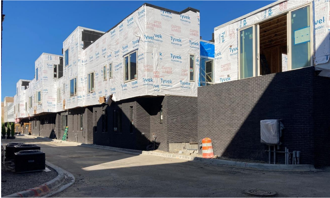
2819-2841 Brush (Carriage House CH4), current appearance
