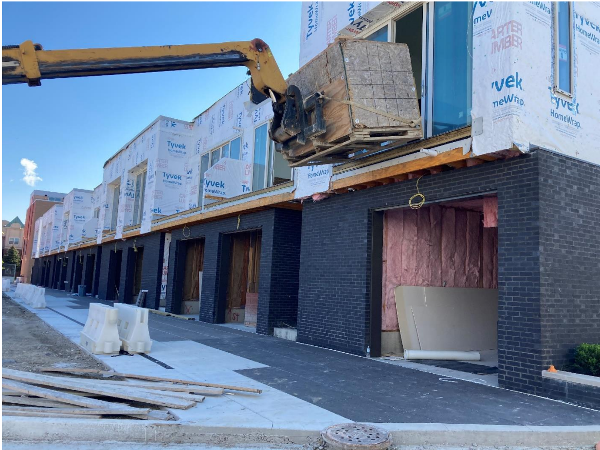
2819-2841 Brush (Carriage House CH4), current appearance
