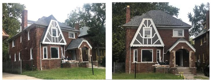
4260 Fullerton. HDC Staff photo – September 14, 2021 – Routine site visit by staff as part of the application and staff reporting process. Note window replacement, roof replacement, front door replacement, metal railing removal. Additionally, staff observed the painting of the front stucco & half-timbering which is additional work that has happened since May without approval from the HDC.
