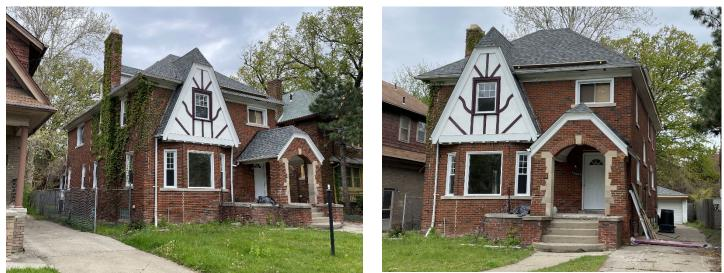
4260 Fullerton. HDC Staff photo – May 10, 2021 – Site visit based on reported violation of work being done without approval. Note window replacement, roof replacement, front door replacement, metal railing removal.
