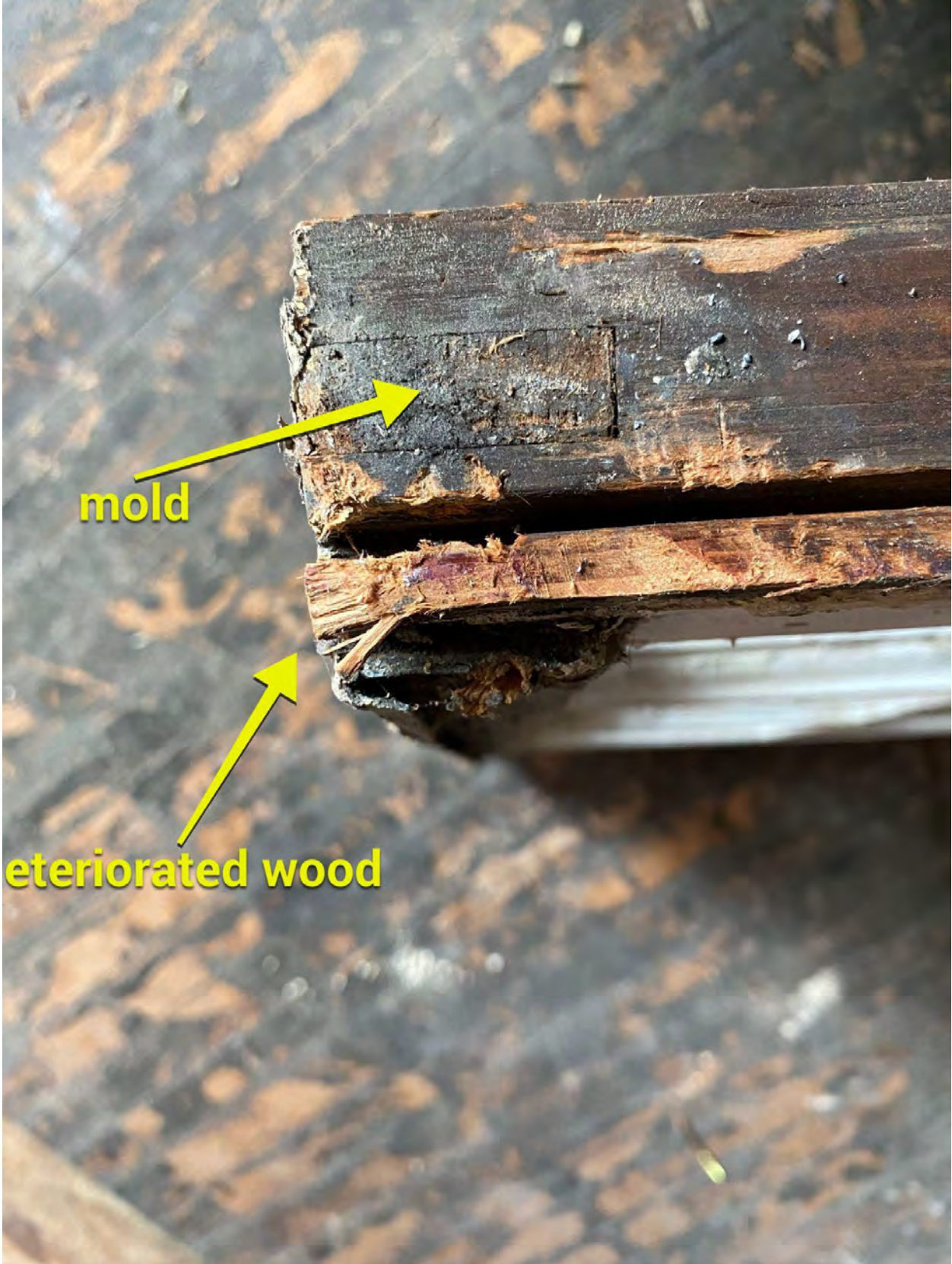
Window 4, 9/1 divided light South Elevation - Right Sash
