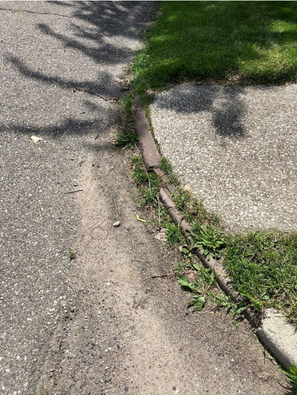
4200 block, masonry curb
