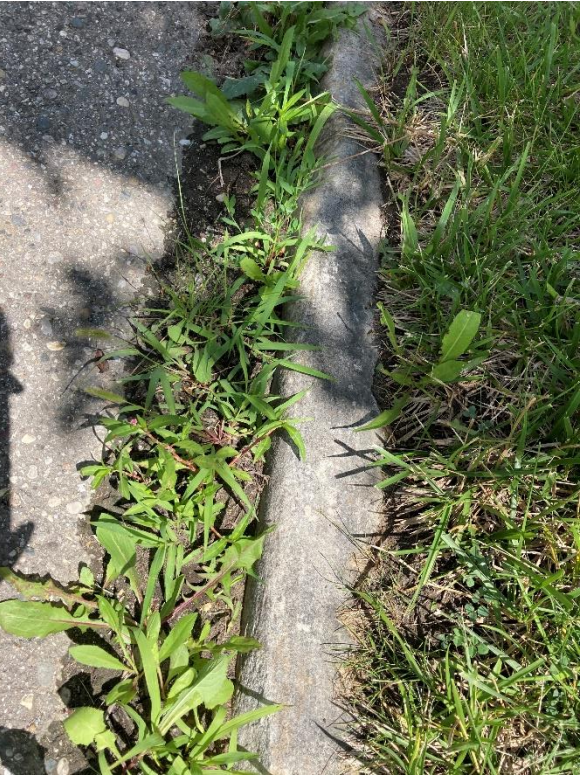
4100 block, limestone curb detail
