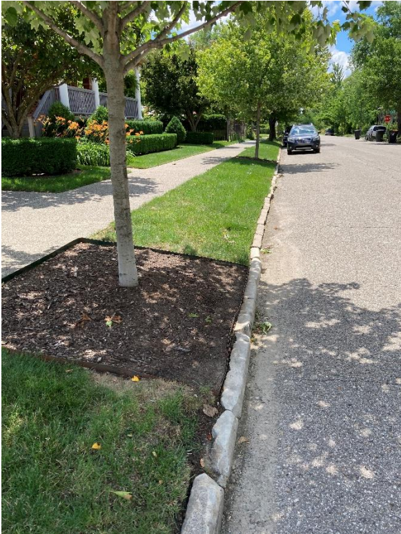
4200 block, concrete curb
