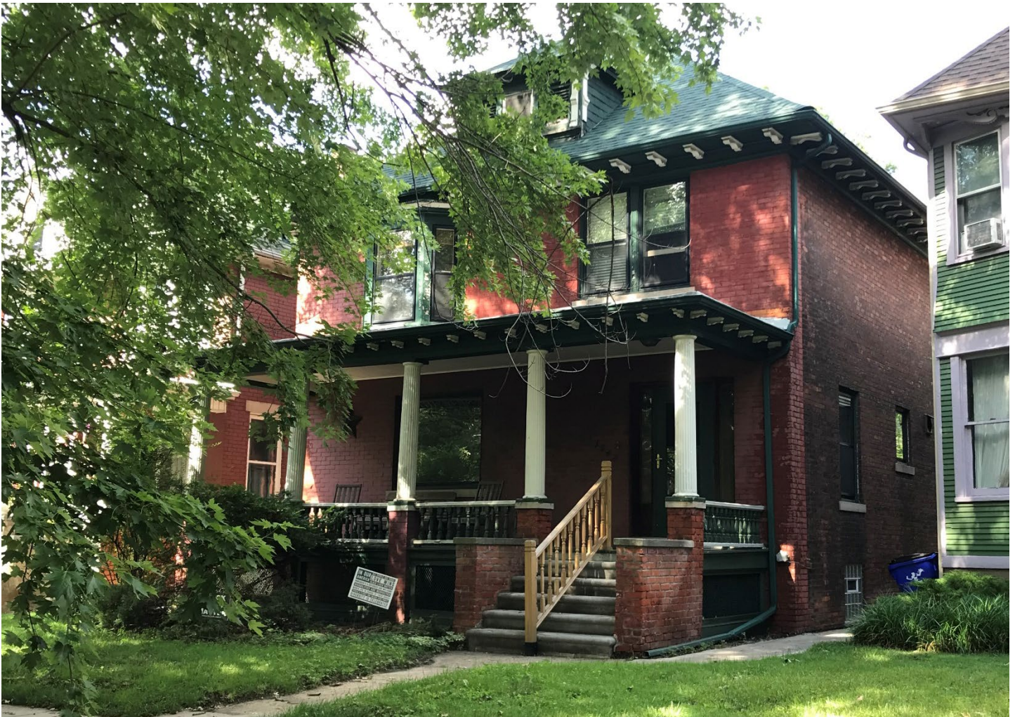
1542 Hubbard. View from Hubbard Street looking northeast. Photo taken by HDC staff, June 28, 2021.
