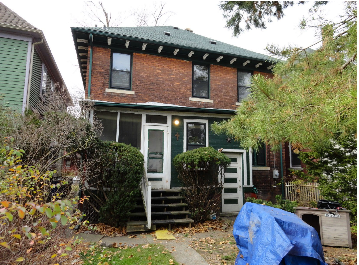
1542 Hubbard. View of existing conditions at rear, looking southwest. Applicant photo.
