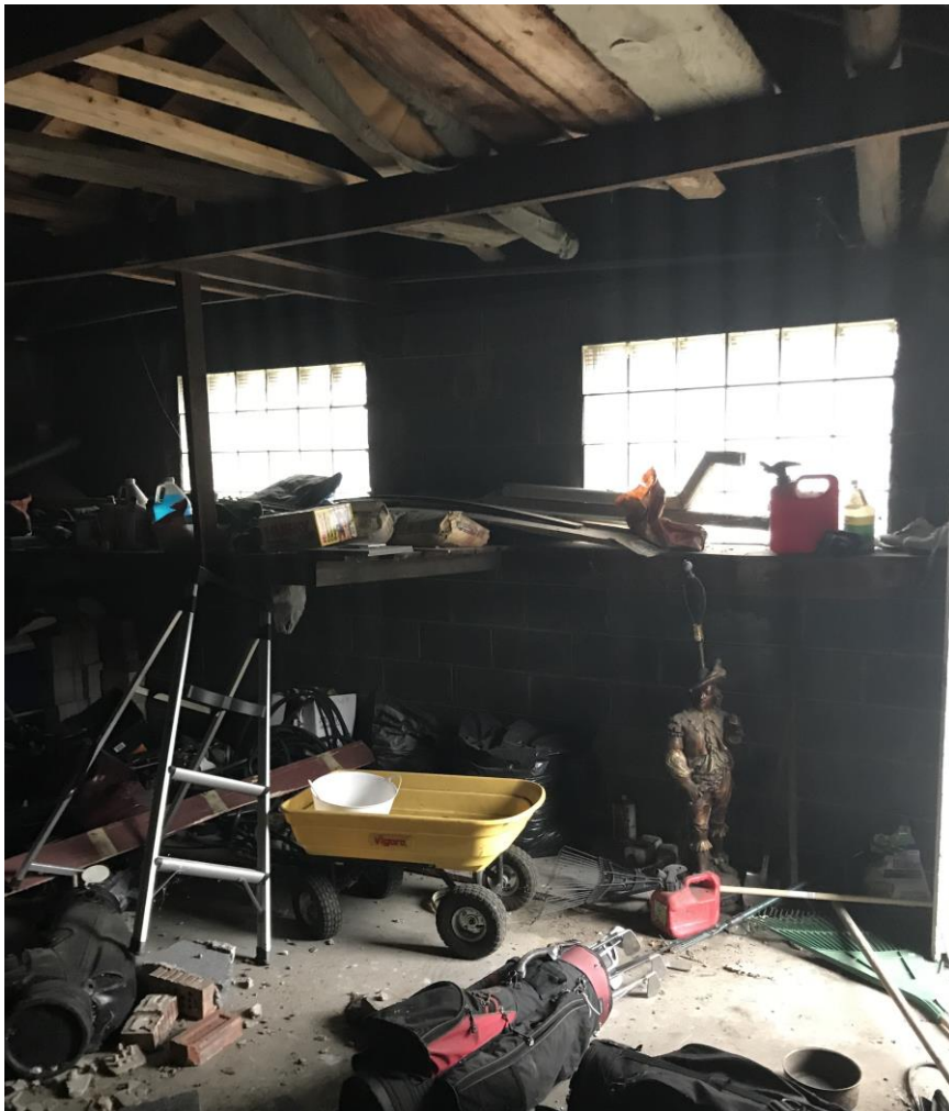
Interior of front/west elevation
