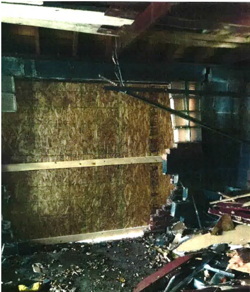
Description of existing conditions-14854 Ashton Rd.
