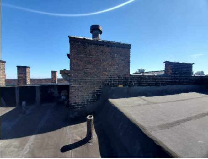
South Elevation of Structure to be Replaced
