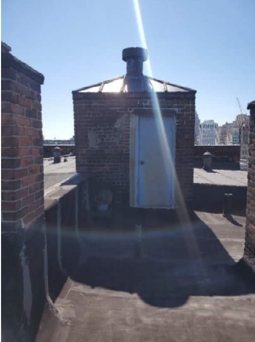
West Elevation of Structure to be Replaced
