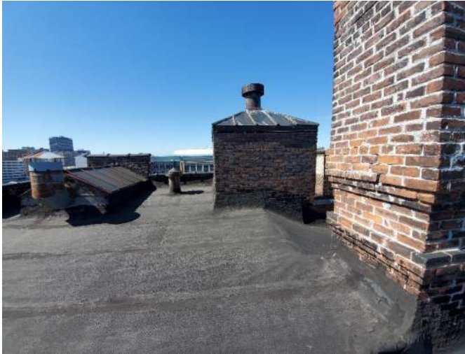
North Elevation of Structure to be Replaced
