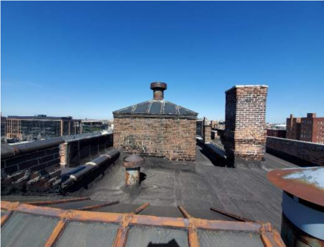
East Elevation of Structure to be Replaced
