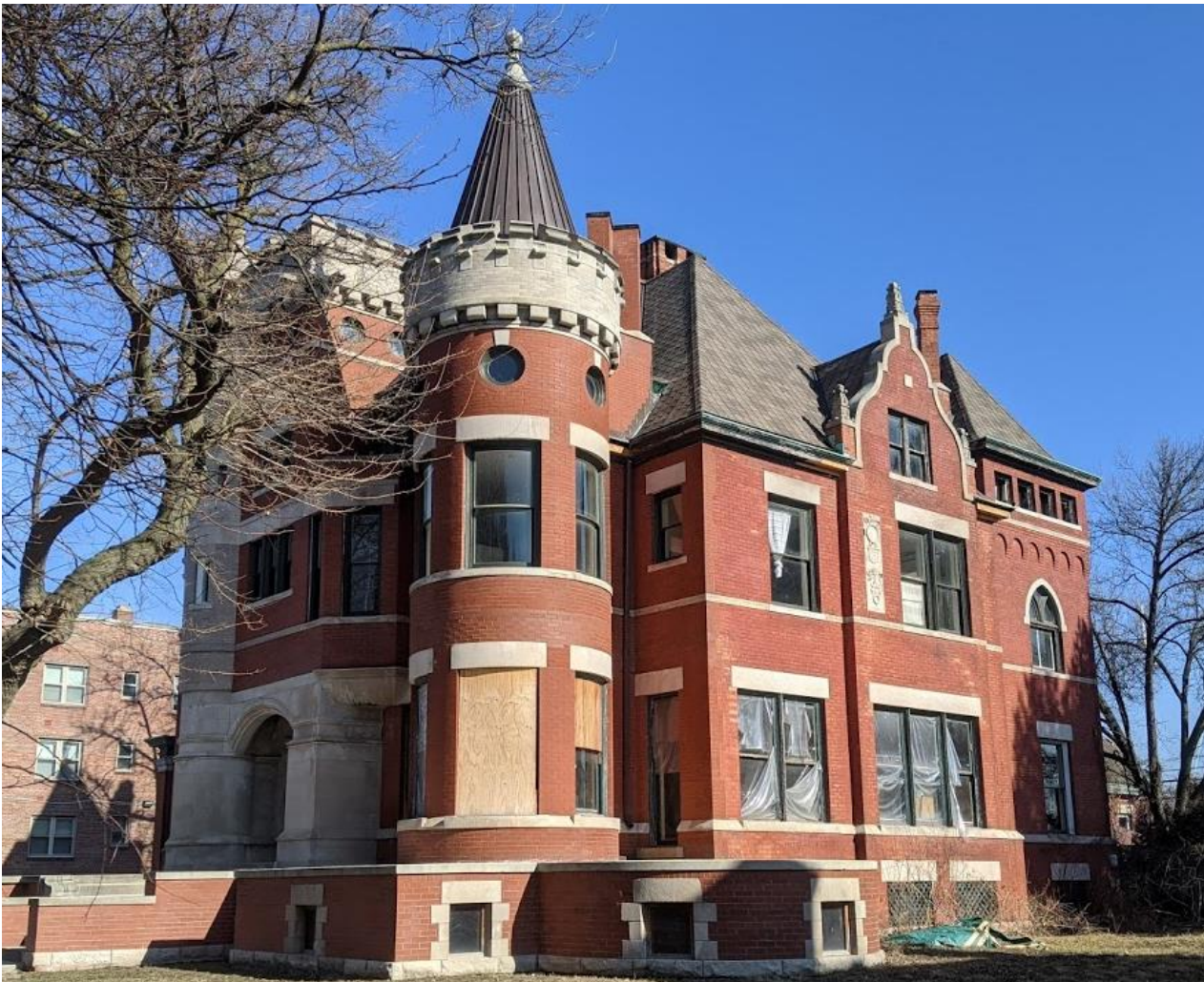
530 Parkview. Note, newer asphalt shingle roof
