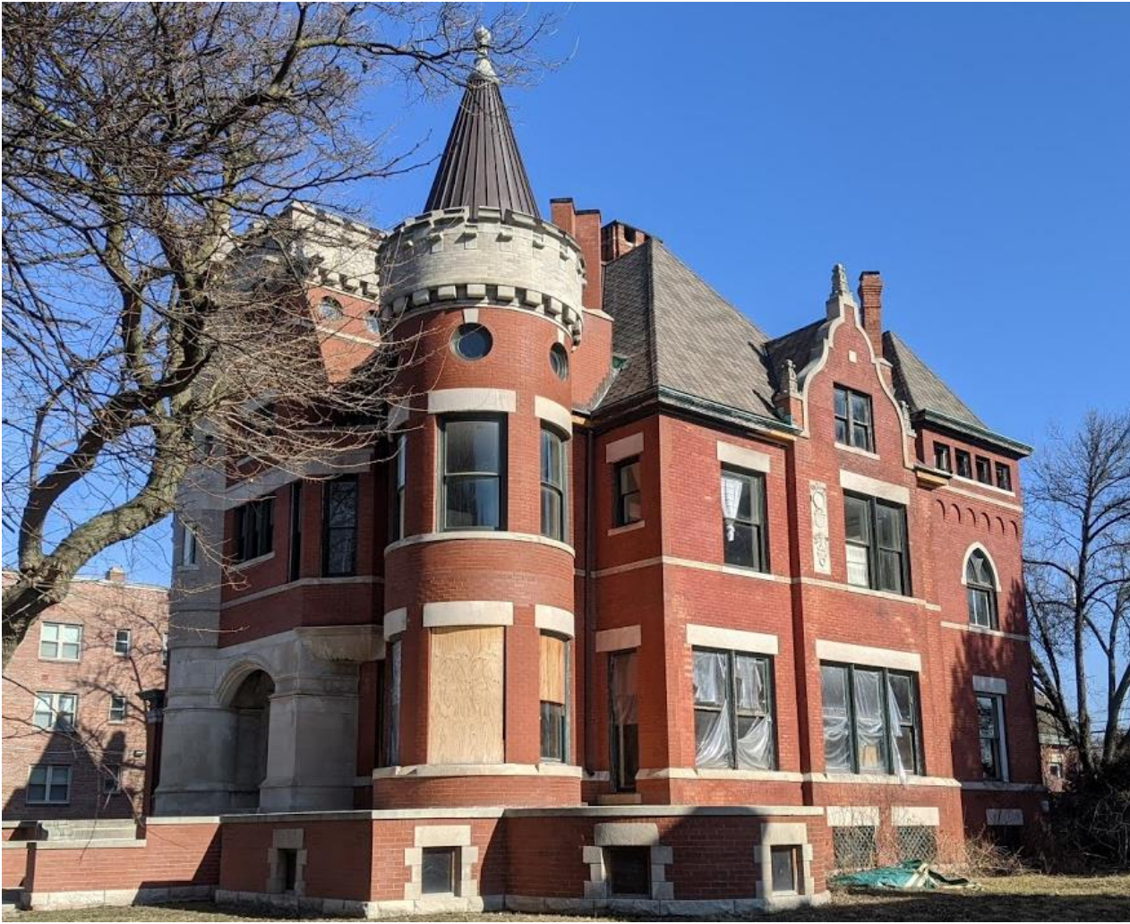
530 Parkview. Note, newer asphalt shingle roof
