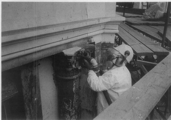
*Figure 11. New methods are being developed or adapted to safely remove lead-based paint from various substrates. On this cast iron building undergoing rehabilitation for apartment units, multiple layers of lead-based paint were removed with pneumatic needle guns with vacuum attachments. Paint chips and waste containing lead-based paint were placed in 55 gallon drums for transport to a special waste site, and the workers were fully protected. The cleaned metal was primed and repainted.*
