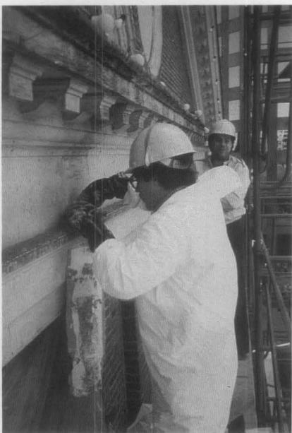
*Figure 10. The choice of paint removal method will trigger various environmental controls and worker protection. The chemical poultice-type paint remover uses a paper backing that keeps the lead waste contained for proper disposal. The worker is adequately protected by a suit and gloves; for this work a respirator was not required. Local laws required containment and neutralization of any after-wash water run off.*
