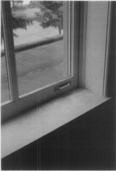
*Figure 22. Research has shown that some small children will chew on projecting window sills while teething. As part of a lead hazard control project, the edge of the sill can be stripped to bare wood or an encapsulating paint applied. In this case, a new window sill was installed as part of a window upgrade that retained the historic trim and frame.*
