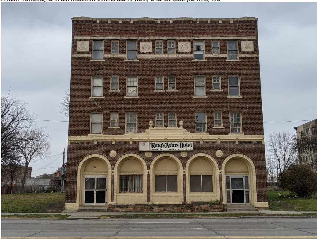
Front elevation view of the King's Arms Hotel (former Hotel Stimson), looking north. Staff photo, December 4, 2020.
