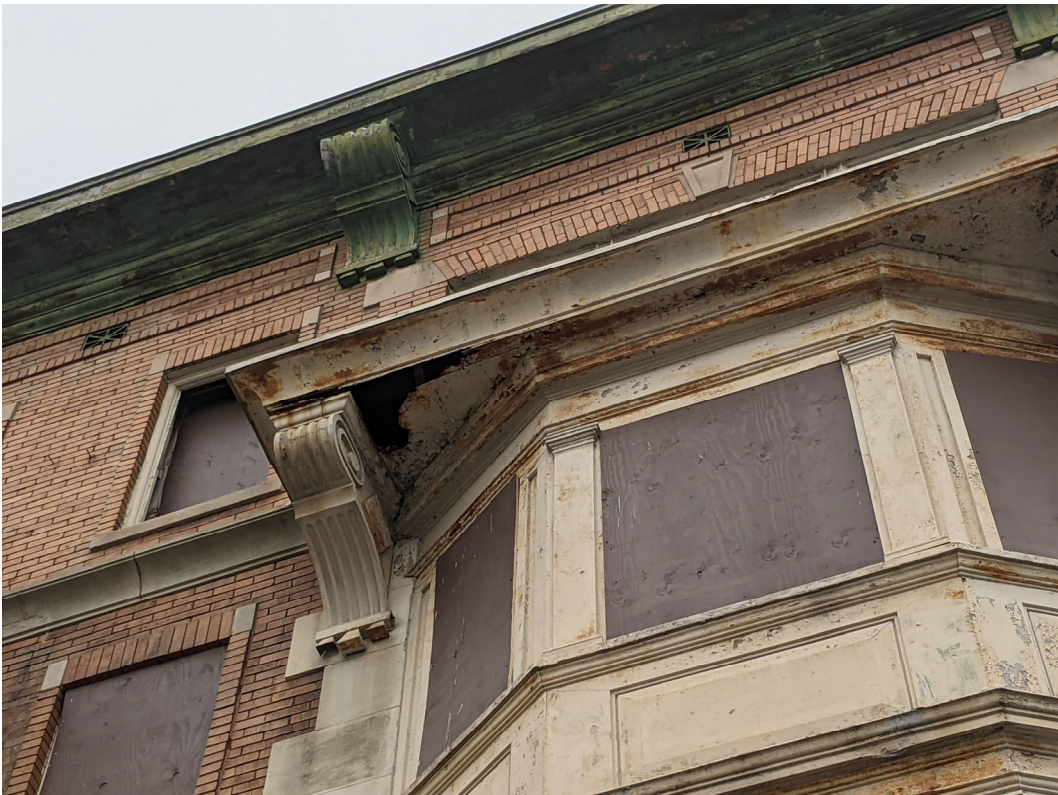
Detail view of metal detailing at bays and cornice, Cass elevation. Staff photo, December 7, 2020.
