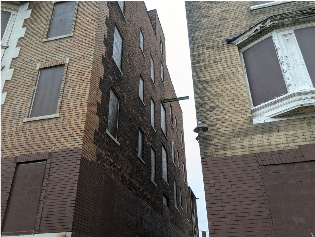
View of northwest corner of building along Henry Street, showing furniture hoist beam projecting from Side (west) elevation, and adjacent 427 Henry building. Staff photo, December 7, 2020.
