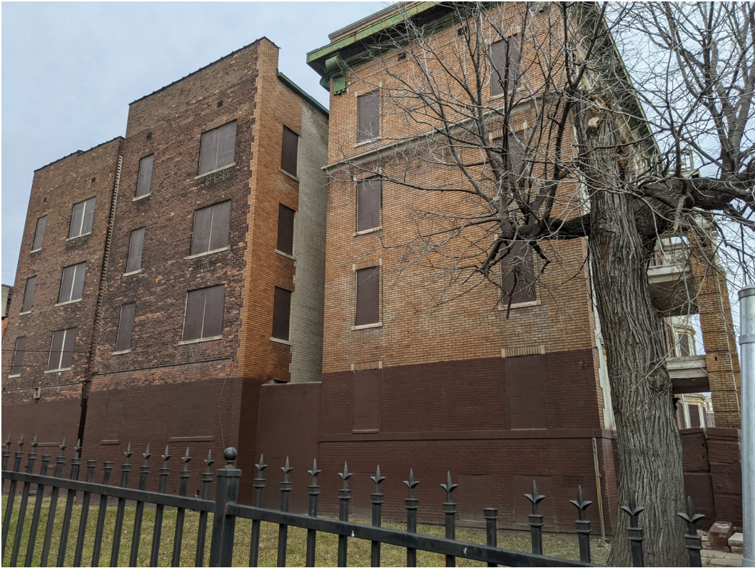
South elevation. Staff photo, November 24, 2020.
