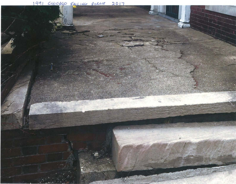
Front Porch Detail (BEFORE) 2017
