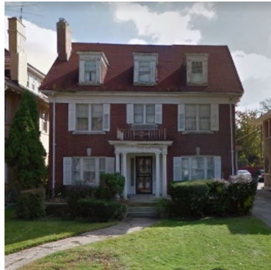
Site Photo 2 by Google Oct. 2014, condition prior to unapproved porch removal
