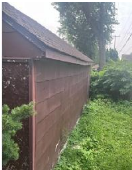
Rear (west wall), looking south towards Chalfonte
