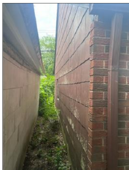
Side (south wall), looking towards rear of property
