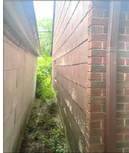
Partial view of brick cladding east wall of garage, at south-side wall.
