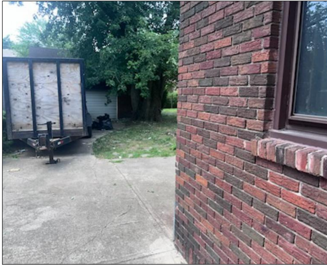
Partial view of south wall of house, looking toward the garage.
