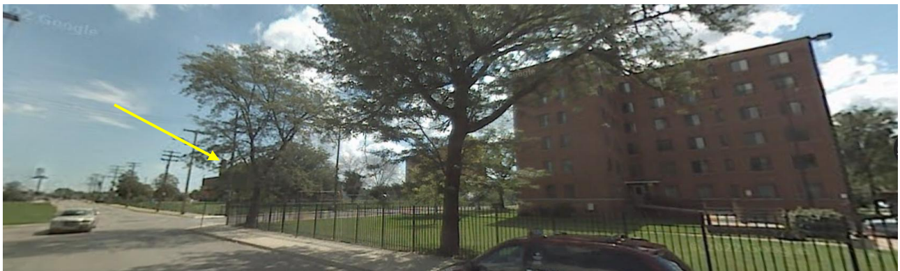
Brewster-Wheeler Recreation Center, 2007 (yellow arrow), with the new demolished Frederick Douglass Apartments to the right/west. Note perimeter fencing. Google Streetview
