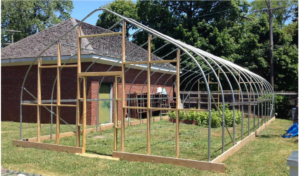
Photo of the hoophouse framing without the plastic sheeting, from applicant's materials.
