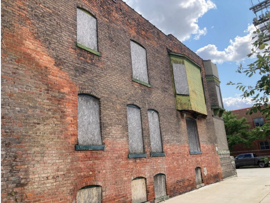
Staff photo, July 2026 shows the north wall, along the alley. These arched openings are to receive rectangular windows, and some of these openings are proposed to be reduced. Additionally, the bay window shown on the red brick portion of the wall is proposed for removal.
