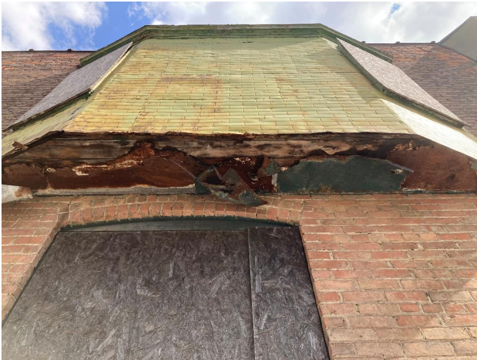
The bay window on the north wall, along the alley, (from below) that is proposed for removal. It is currently covered in metal siding that looks like brick. (Staff photo, July 2026)
