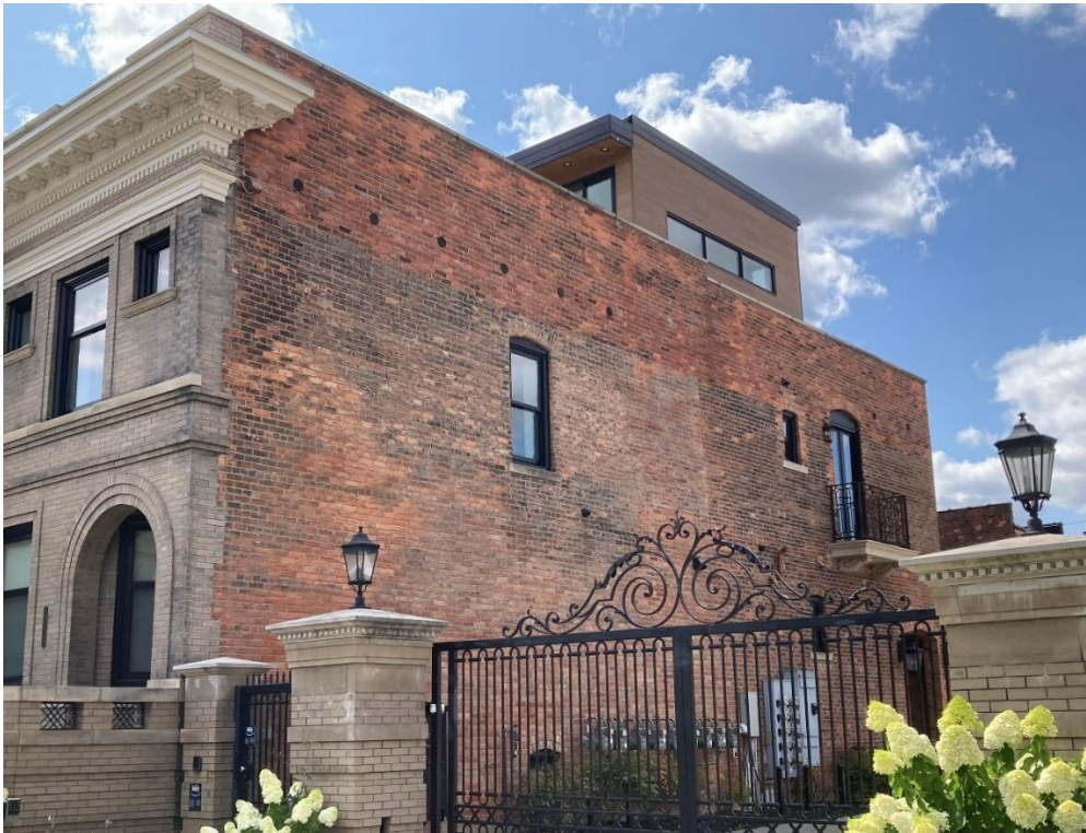
Staff photo, July 2026, shows replaced windows and doors that are rectangular units in rounded openings on the east side of the rehabilitated units on Erskine, south of the scope area. On these secondary, red-brick elevations, staff does not find that these rectangular units in rounded openings diminish the building's historic character.
