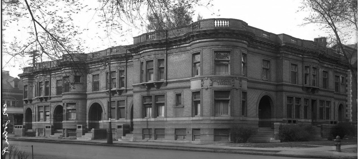
Undated, historic photo of Patterson Terrace Apartments from PDD’s files. The John R units proposed for rehabilitation are the three units furthest to the left of this image. The fourth John R unit’s doorway (3412 John R) is barely visible here behind the Erskine units, shown to the right of the image. Visible are the building’s cornices and balustrades and cottage-style windows with the upper sashes shorter than the lower.
