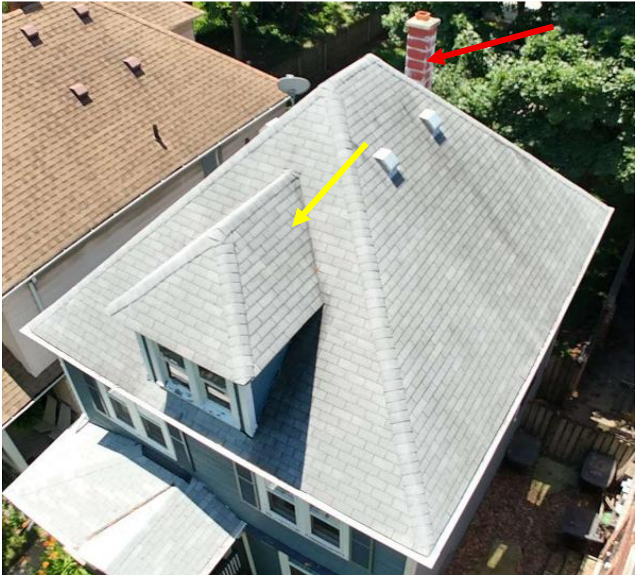
Photo of existing roof. Note hipped roof dormer at the front façade (yellow arrow) roof surface and chimney at rear which is proposed for removal (red arrow). Photo by applicant
