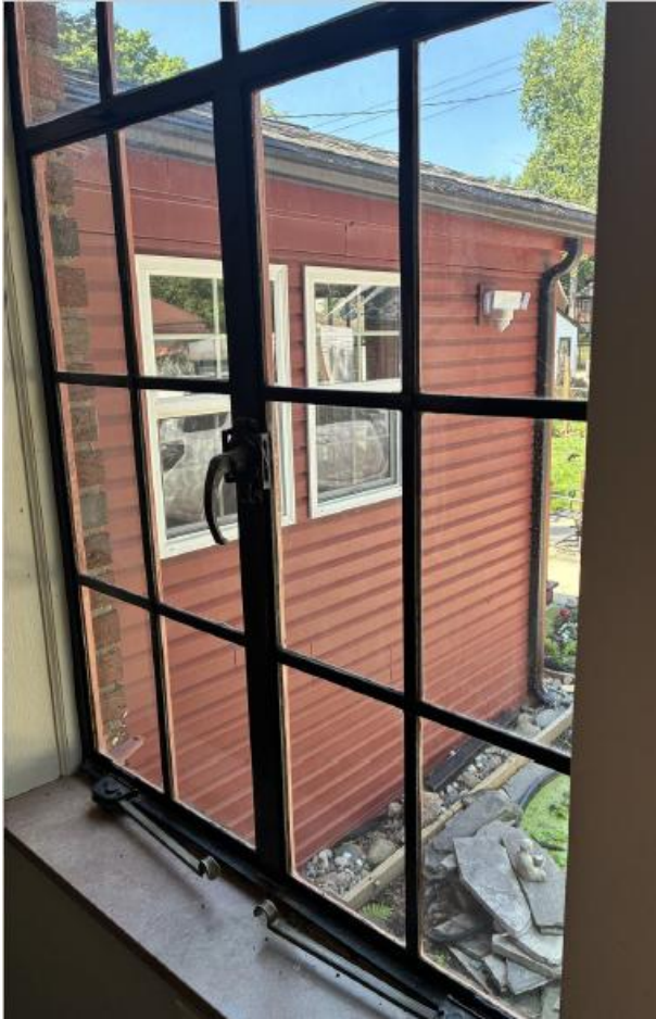
Applicant photo of the paired casements in the bay window. Proposed is a fixed window.
