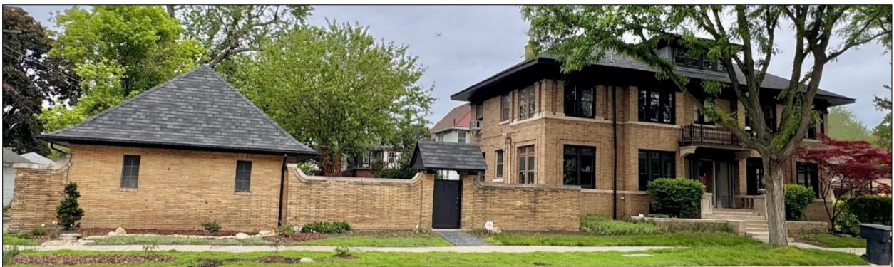
801 Edison rear yard masonry wall enclosure. View from 3 rd Avenue, looking west. Staff photo, 05/20/2026.
