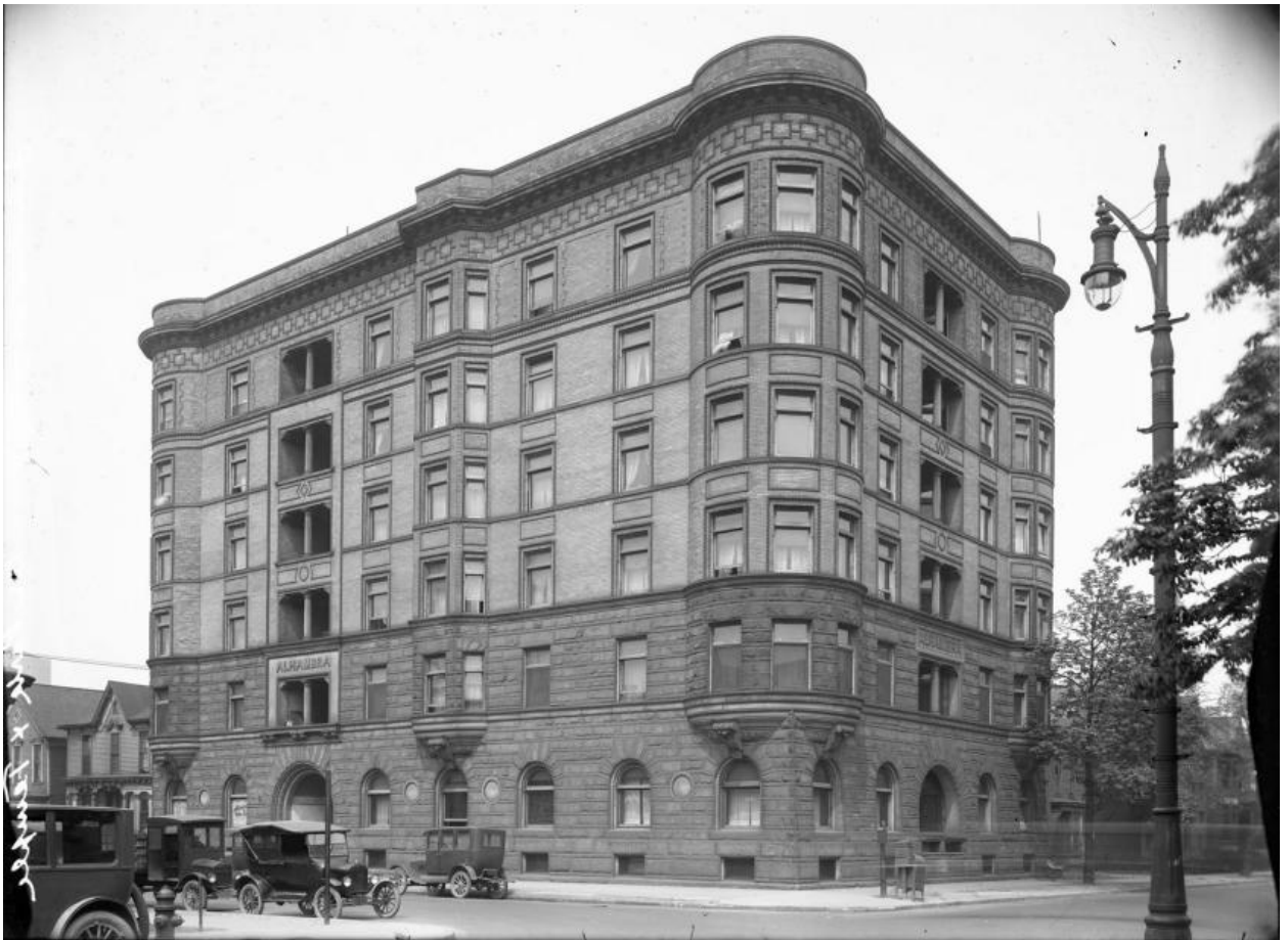
1920s photo from applicant's materials. The long, south side along Temple is shown, along with the short, east end along Park. Fire escapes were added to the Park Avenue façade by the 1970s. A building permit to add a counterbalanced fire escape system to the building was issued in 1940.
