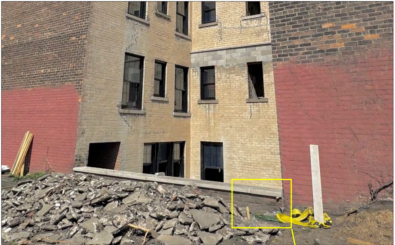
Central lightwell. The new retaining wall is clad with at least four courses of brick. Staff photo, 04/22/2026.
