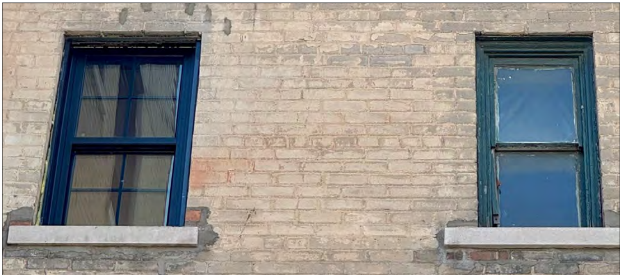
Staff photos of wood and replacement windows on the east side, central courtyard/lightwell. The dimensionality of the historic brickmold is visible, in comparison to the flat, thin trim installed against the replacement window. The importance of wood brickmold is clear: the window retains a highly dimensional appearance (even with a 1-over-1 pattern) in comparison with the 6-over-6 internal grid replacement window. 04/22/2026
