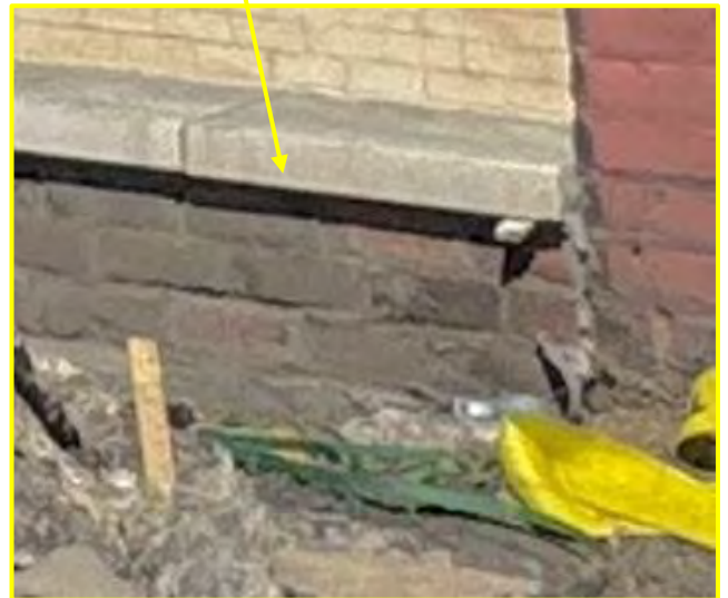
Central lightwell. The new retaining wall is clad with at least four courses of brick. Staff photo, 04/22/2026.
