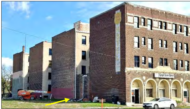
Full west side of building. Staff photo, 04/30/2026.
