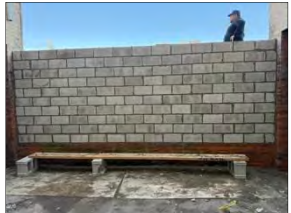
Above and below: Undated applicant photos. Below is an interior wall view of a newly constructed wall, extending into a retaining wall of a lightwell prior to the installation of cast stone.
