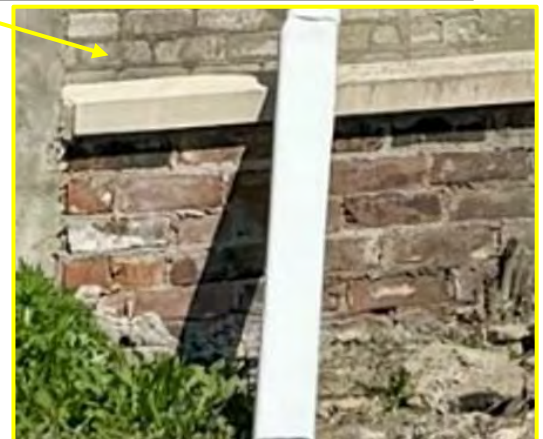
Rear lightwell. The new retaining wall is clad with five-to-six courses of brick. Current grade is substantiated by the remaining grass at the base of the outer building walls. Staff photo, 04/22/2026.
