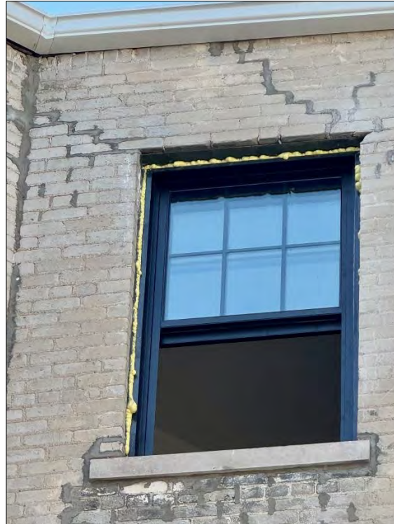
Staff photos of wood and replacement windows on the east side, central courtyard/lightwell. The dimensionality of the historic brickmold is visible, in comparison to the flat, thin trim installed against the replacement window. The importance of wood brickmold is clear: the window retains a highly dimensional appearance (even with a 1-over-1 pattern) in comparison with the 6-over-6 internal grid replacement window. 04/22/2026
