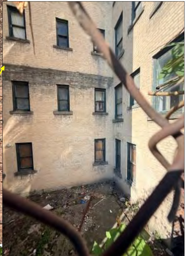
Undated applicant photo of the east side central lightwell prior to work taking place. The brick that was replaced with CMU is visible, as is the chain link fencing that previously enclosed these recessed openings.
