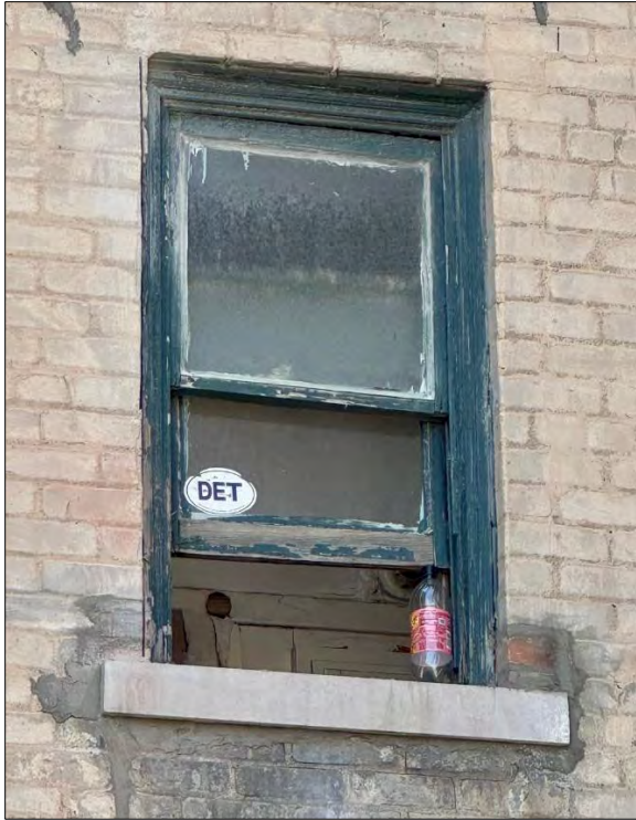
Staff photos of wood and replacement windows on the east side, central courtyard/lightwell. The dimensionality of the historic brickmold is visible, in comparison to the flat, thin trim installed against the replacement window. The importance of wood brickmold is clear: the window retains a highly dimensional appearance (even with a 1-over-1 pattern) in comparison with the 6-over-6 internal grid replacement window. 04/22/2026
