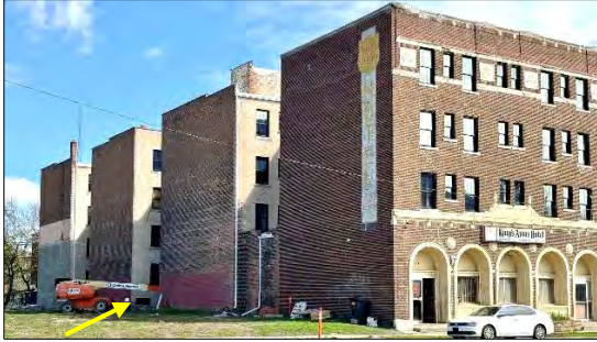
Full west side of building. Staff photo, 04/30/2026.
