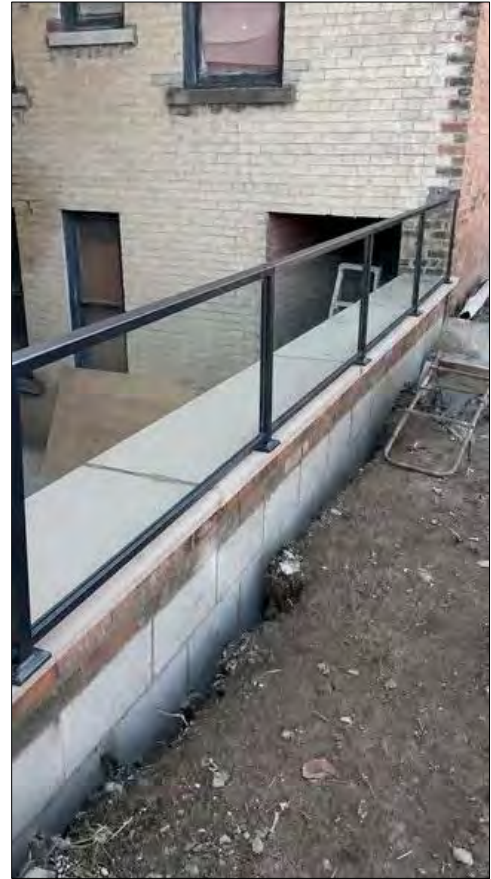
Above and below: Undated applicant photos. Below is an interior wall view of a newly constructed wall, extending into a retaining wall of a lightwell prior to the installation of cast stone.
