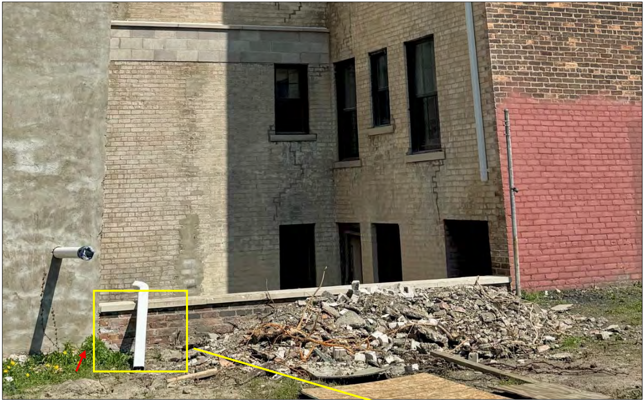
Rear lightwell. The new retaining wall is clad with five-to-six courses of brick. Current grade is substantiated by the remaining grass at the base of the outer building walls. Staff photo, 04/22/2026.
