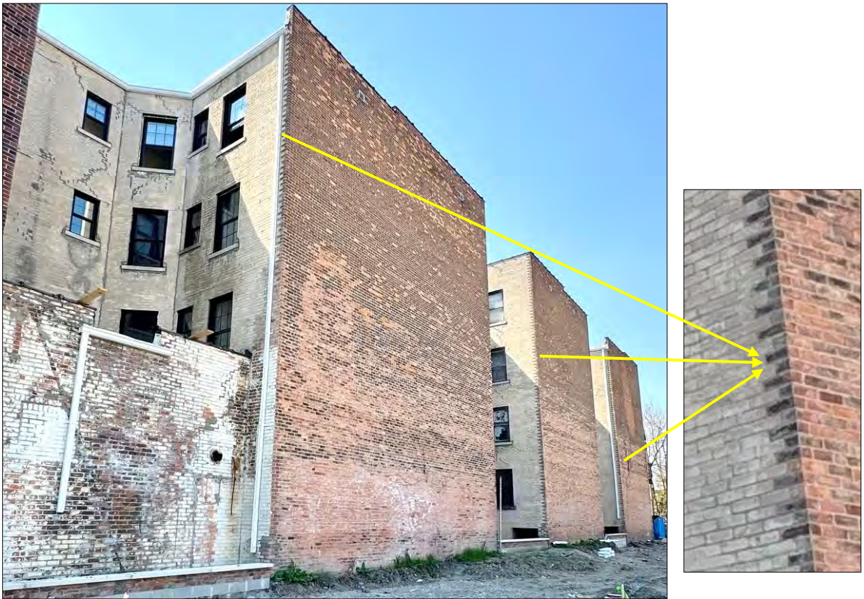
The stepped brick pattern occurs at the interior edge of each corner of the courtyards/lightwells (east and west sides). Staff photo, 04/22/2026.
