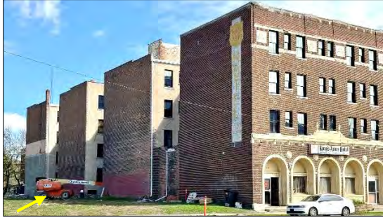
Full west side of building. Staff photo, 04/30/2026.
