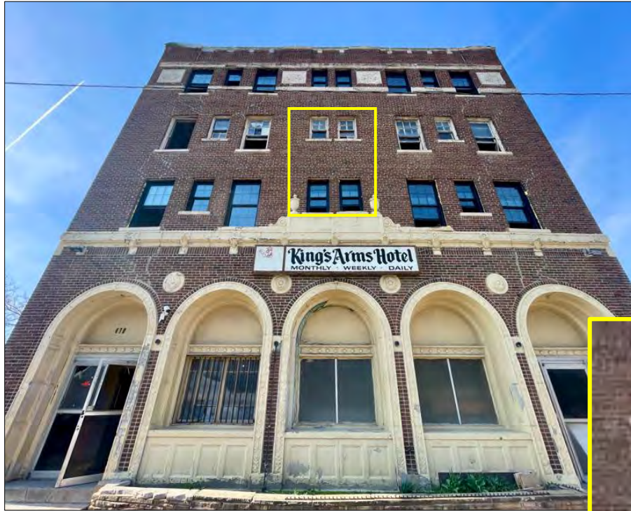
Condition of façade, April 9, 2026. Staff photo.
