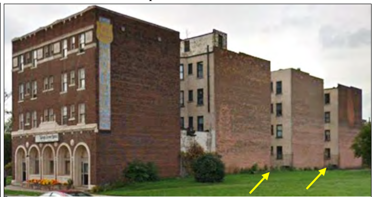
Google Streetview, October 2011. East wall of King's Arms. The four bays are visible due to earlier demolitions of adjacent buildings. You can see the chain link fencing enclosing the central and rear courtyards/lightwells.
