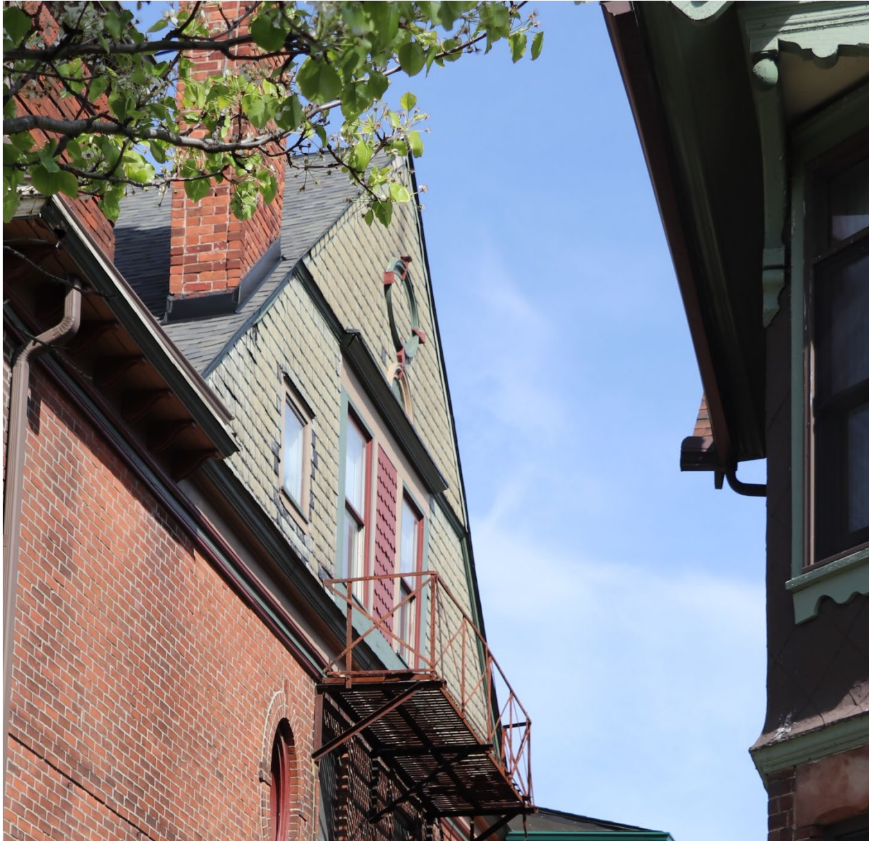
Photos taken by staff 05/04/26 (north-east facing gable end)
