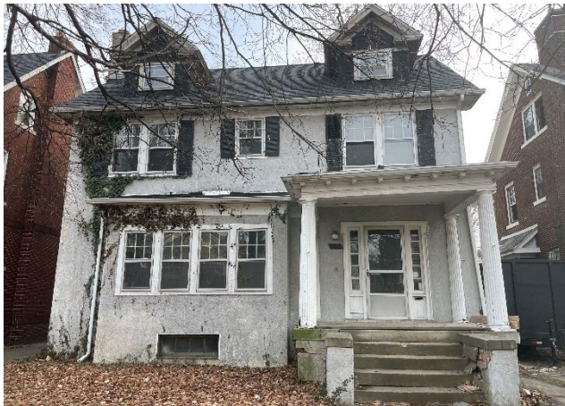
Staff photo taken 12/21/2023 (due to violation)
