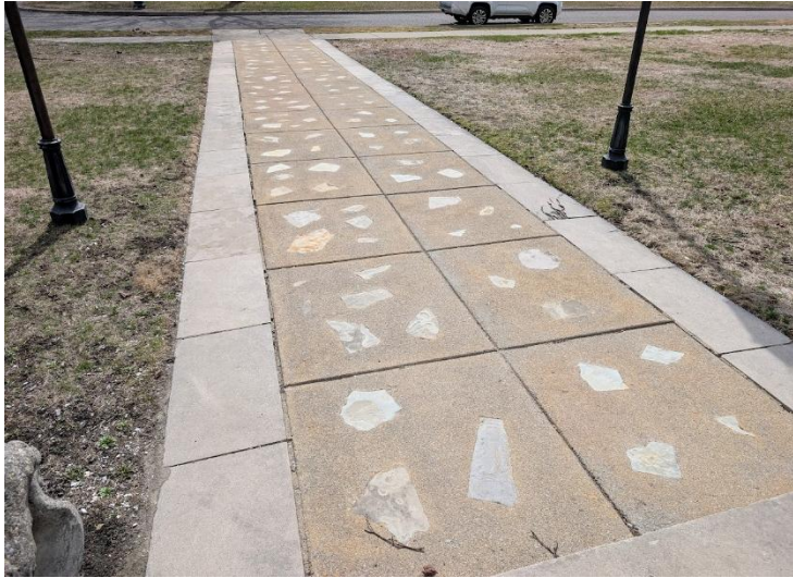
Front walk, current conditions. Insensitive patches are evident. Staff photo, March 2026.
