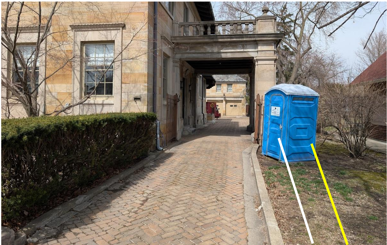
The proposal is to widen the drive along its middle, keeping its beginning point at the sidewalk as it is, adding about 5'8" along the middle, and then curving west toward the porte cochere to add about 2.5' to the end point at the porte cochere. Staff drew a white line roughly where the end point at the porte cochere is proposed, and the yellow line is staff's estimate of where the proposed drive would be at its widest point. (Staff photo, April 2026)
