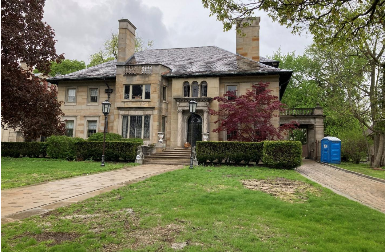
The existing, historic driveway is about 9'6" wide at the sidewalk and remains that width up to the porte cochere, curving westward slightly toward the house to tuck under the porte cochere.
