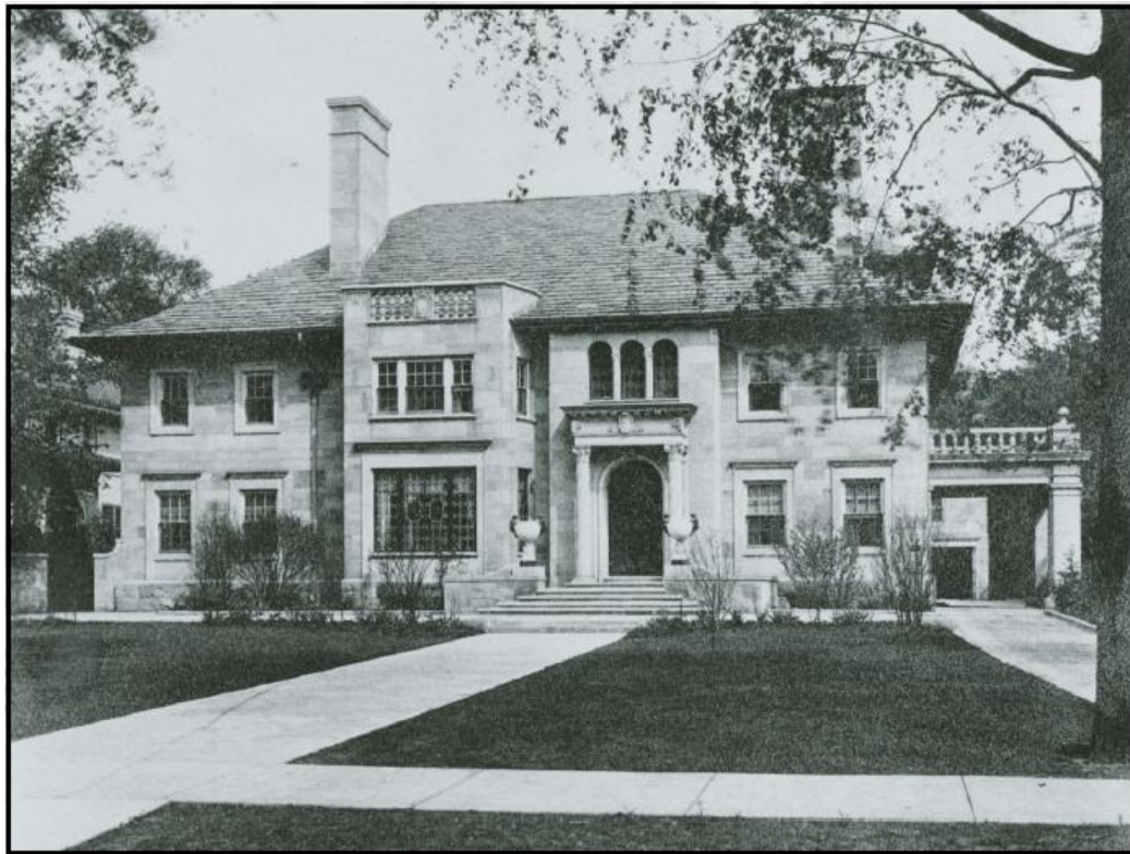
Detail of historic photo above from application materials. It appears to staff that there is a crack in the entry path near the sidewalk, which indicates to staff that this path was concrete and not pavers or bricks (like the drive).
