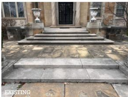
Existing masonry staircases, walls, & piers to remain. Wash and tuckpoint to clean up.
