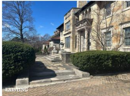
Existing masonry staircases, walls, & piers to remain. Wash and tuckpoint to clean up.
