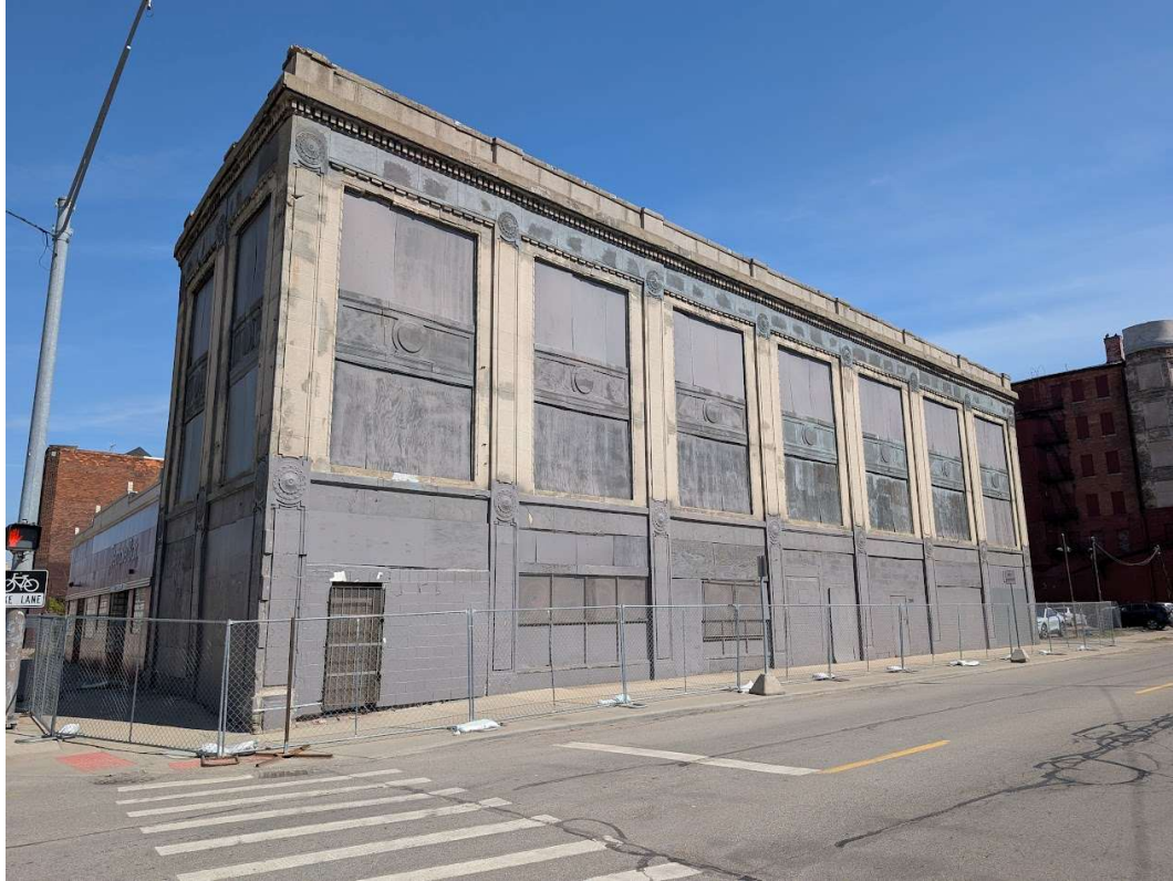
General view of 2900 Cass, looking northwest, fronting Temple Street. Staff photo, April 23, 2026.
