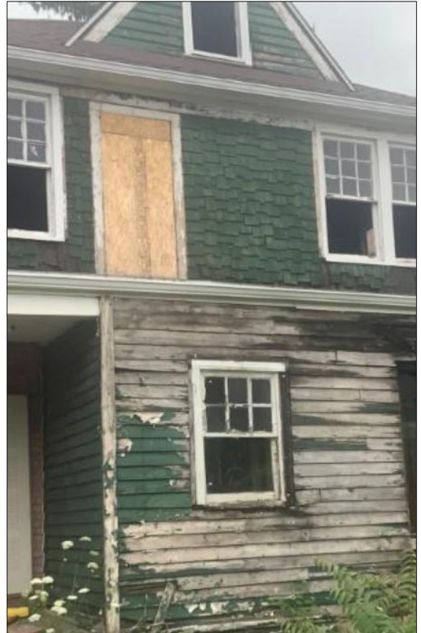
Close-up of applicant photo prior to wall demolition.
