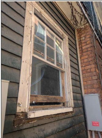
4221 Cortland - Existing 6" Wood Lap Siding (Exposure 4-1/2")
