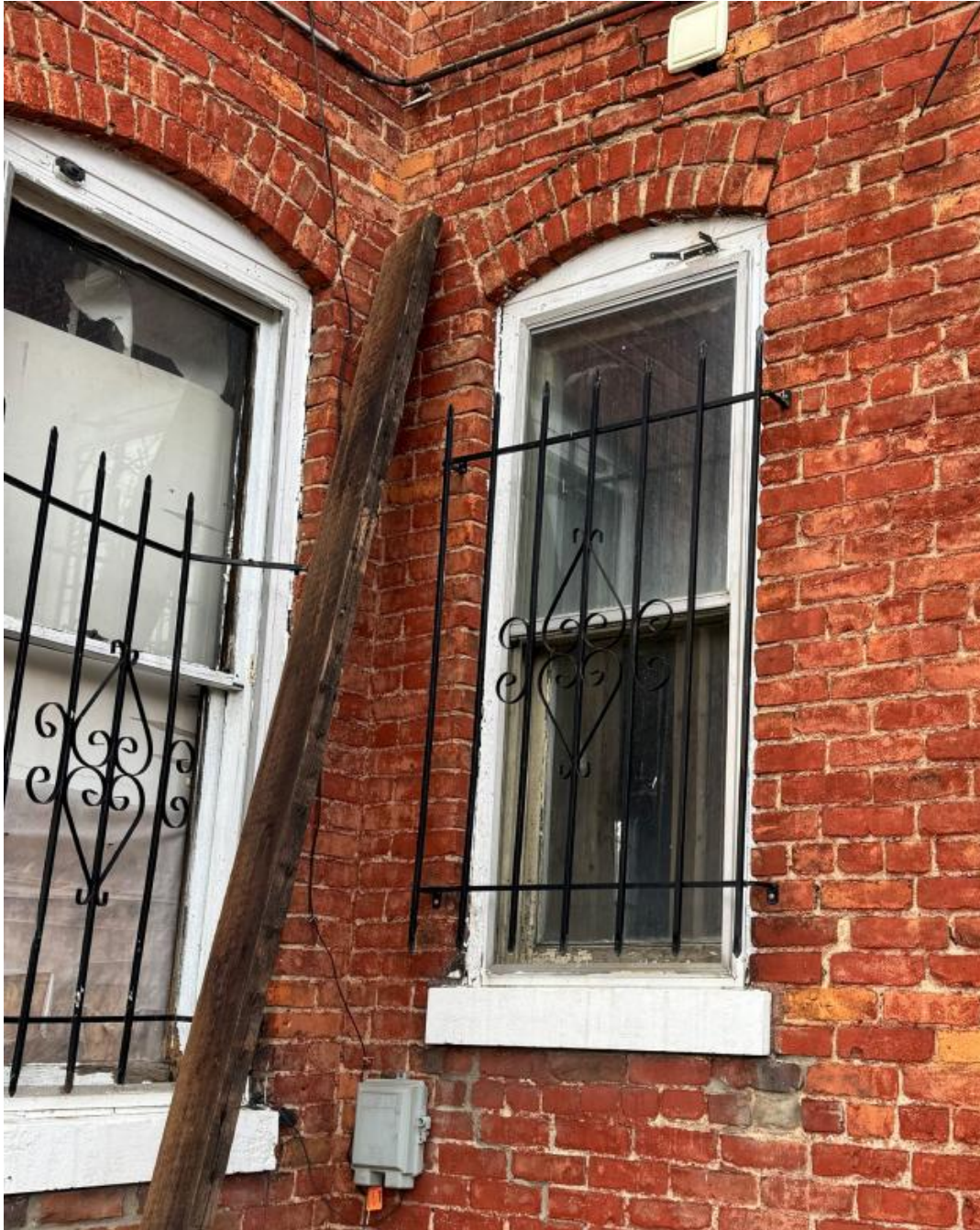
Photo by applicant, showing typical conditions at existing windows
