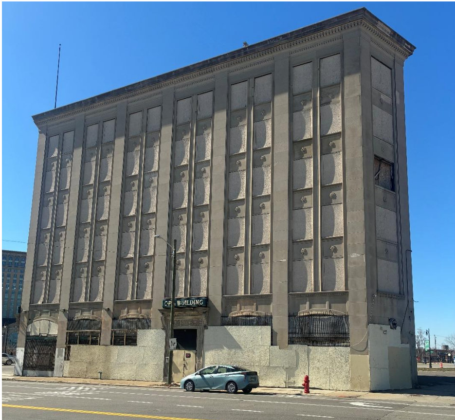
Current appearance. Photo by staff on 03/26/2026. Facing southwest
