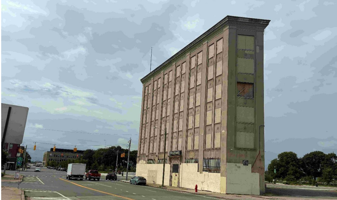
Current appearance. Photo by staff on 03/26/2026. Facing southwest
