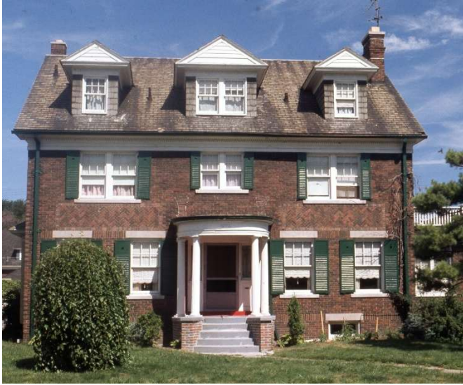
HDAB designation photo, 1974, showing historic windows
