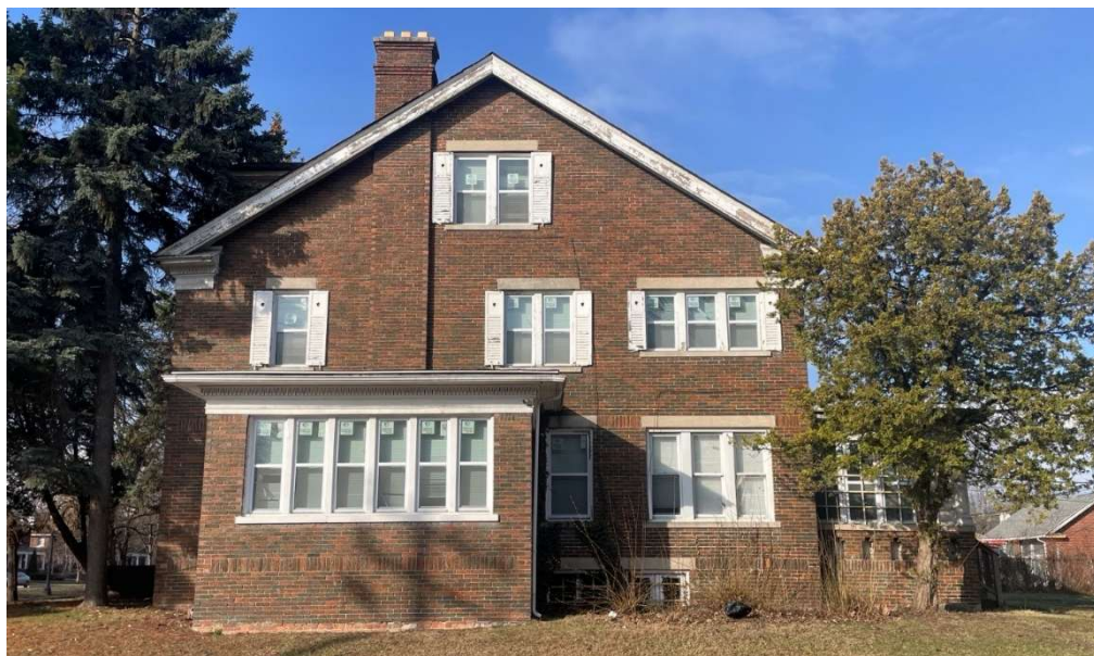
West side of house, staff photo, 03/24/2025, after window replacement
