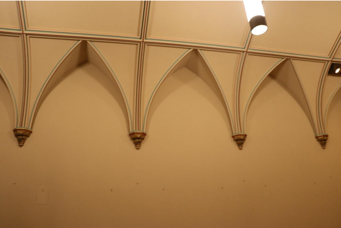
Ceiling detail, Chapel. Photo by staff
