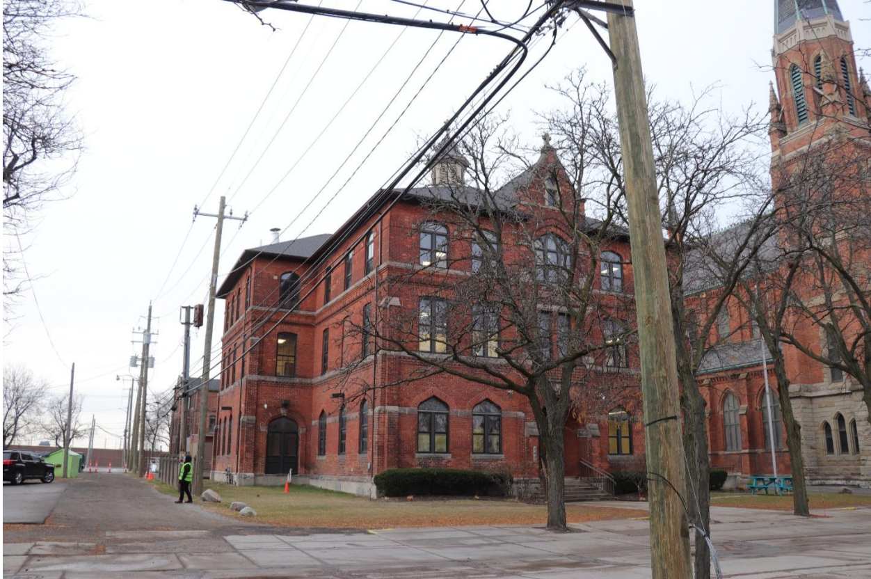
The eastern edge of the historic district is the north-south alley between W Lafayette and Howard Street, shown here from the north looking south. (Staff photo, November 2025)
