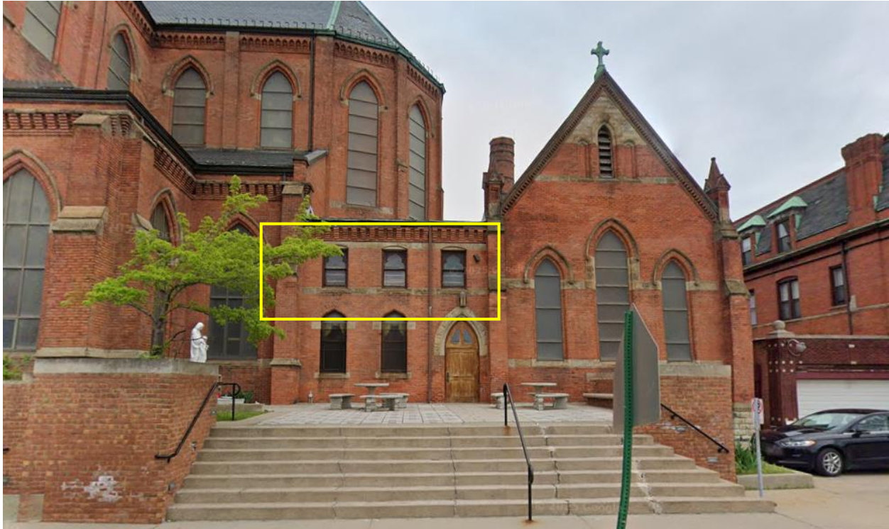
Google Streetview image. Three windows at basilica proposed for replacement, outlined in yellow
