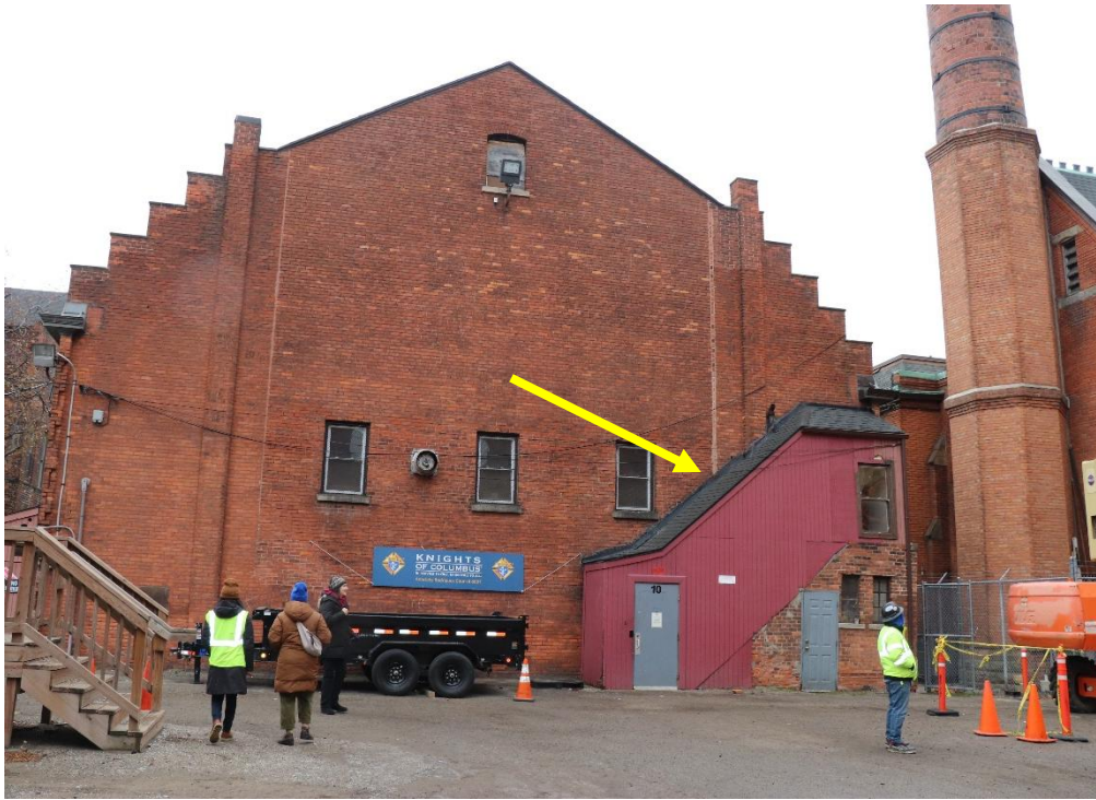
The rear of the Parish Hall, showing the enclosed staircase proposed for removal (yellow arrow). Staff does not find the enclosed staircase to be historic or character defining and does not object to its removal. (Staff photo, November 2025)
