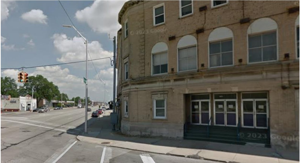
By July 2017, the sign had been removed. (Google Street View) The following year, the local historic district was established.
