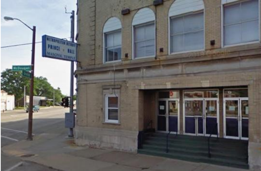
The nonhistoric, illuminated sign was visible at 3500 McDougall in June 2009. (Google Street View)
