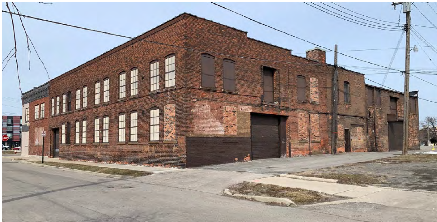
North East view facing on the 10 th street side of the building. *Note portion of the building is from the 1916 addition.
