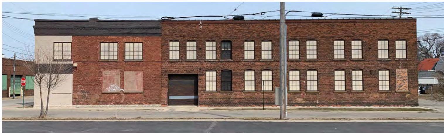
East view facing the 10 th street side of the building. *Note the left section of building is from 1894, where the back portion of the building is from the 1916 addition.
