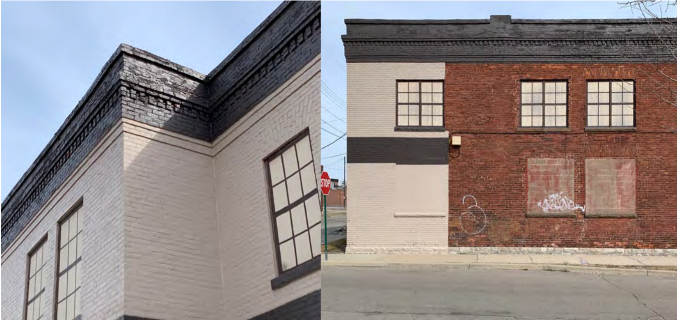
Detail view of historic ornamental cornice brickwork.
