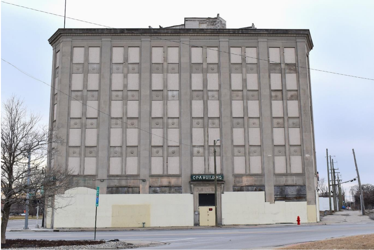
East elevation along 14th St. with partial view of penthouse (February 2025).
