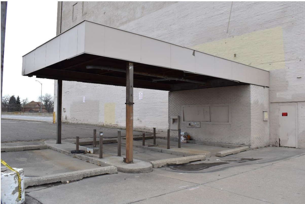
Detail view of non-historic drive-through structure/canopy (February 2025).
