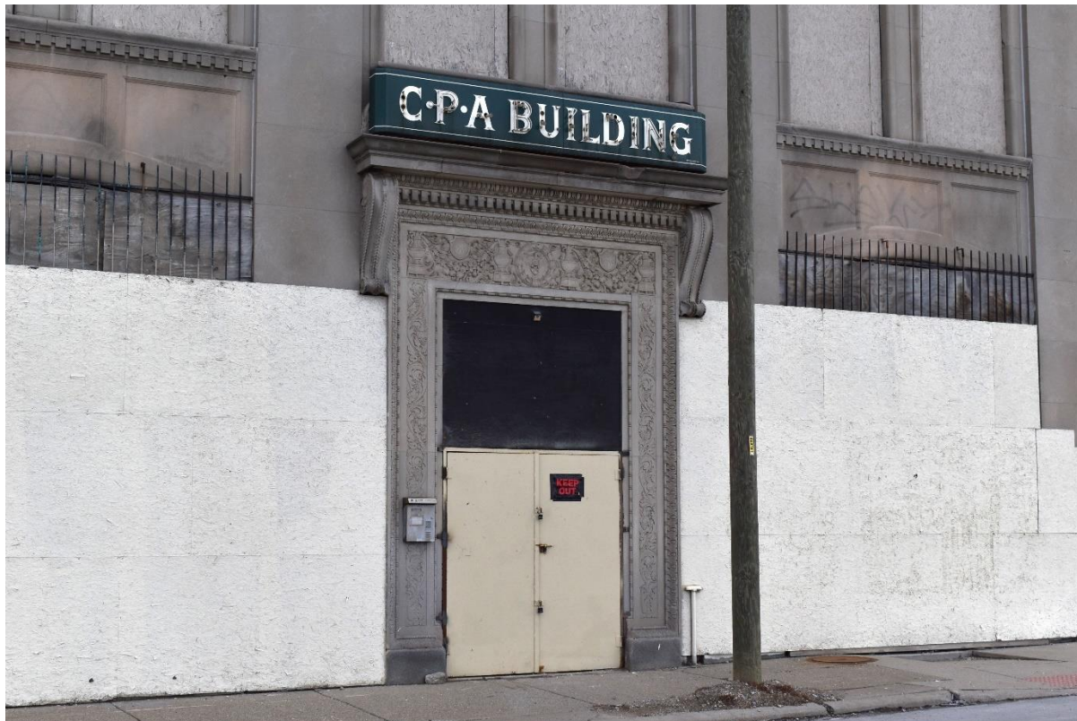
Detail view of secondary entrance along 14th St. (February 2025).
