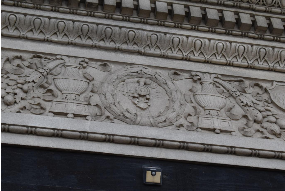
Detail view of carved stonework and locomotive detail above 14th St. entrance (February 2025).
