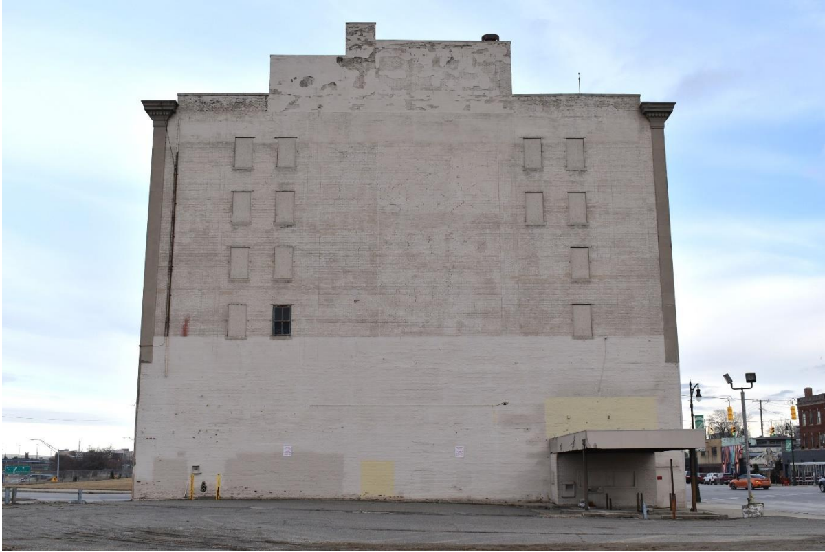
West elevation with partial view of penthouse and drive-through structure/canopy (February 2025).
