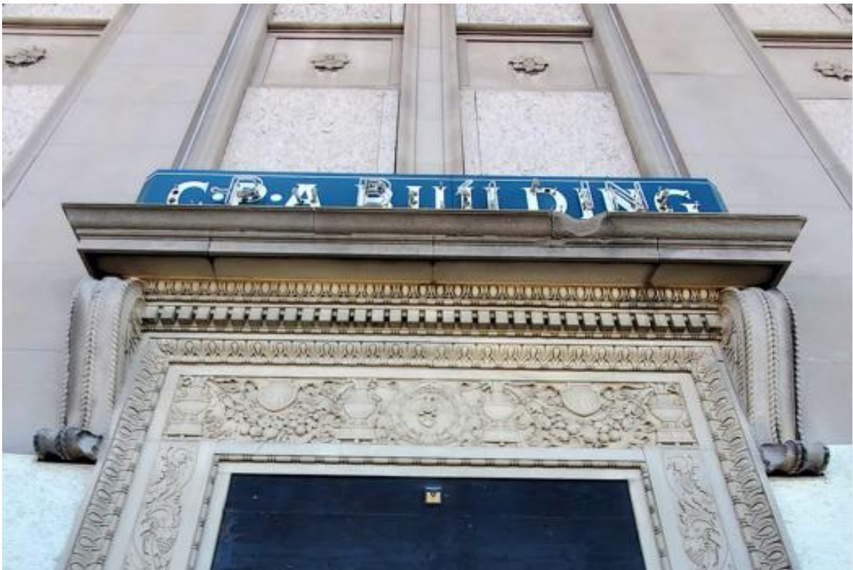
Detail view of carved stonework and sign above 14th St. entrance (November 2025).
