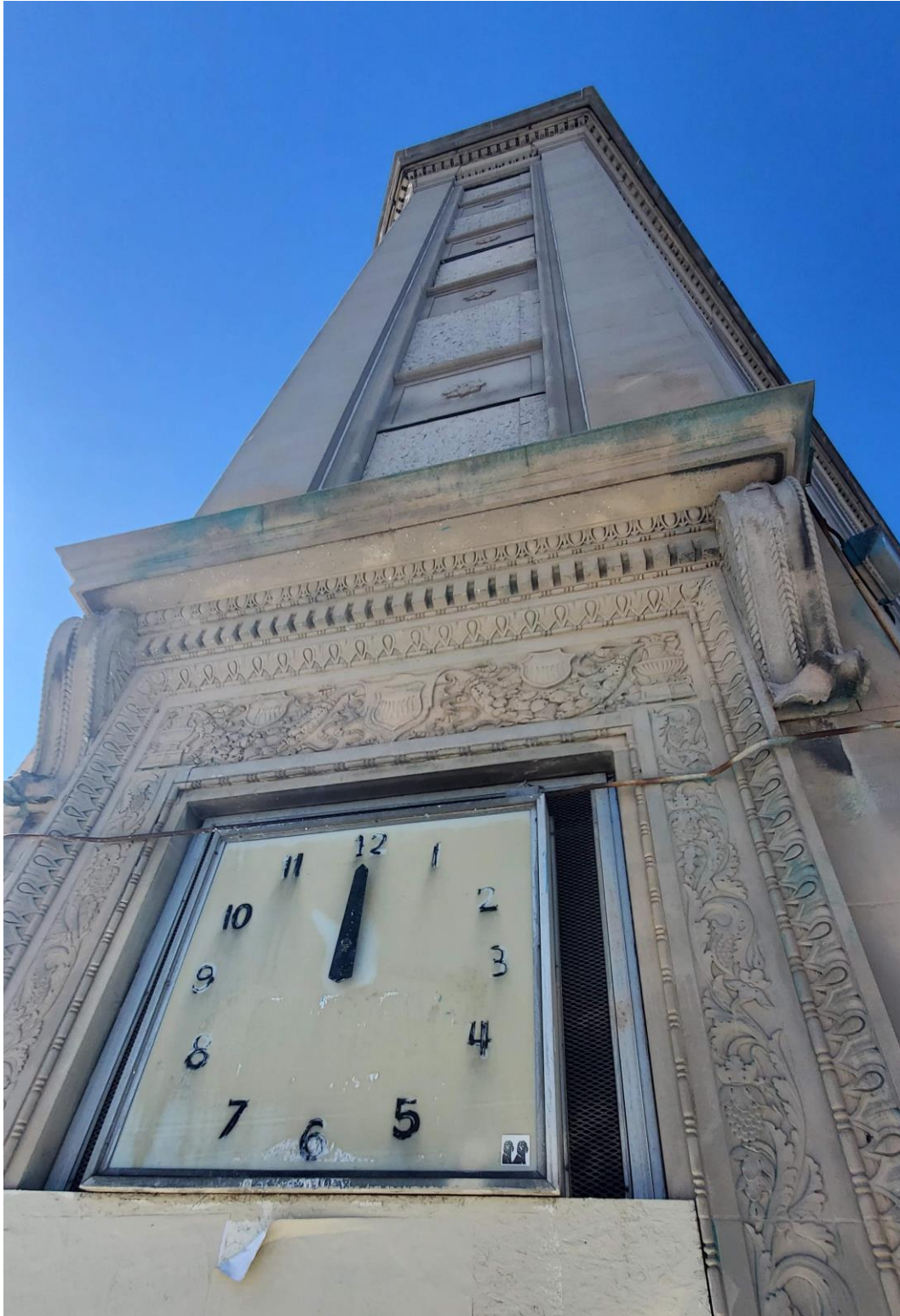
Main entrance at corner of Michigan Ave. and 14th St., architectural details and non-historic replacement clock (November 2024).
