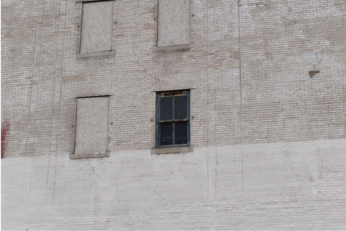
Detail view of original window on west elevation (February 2025).
