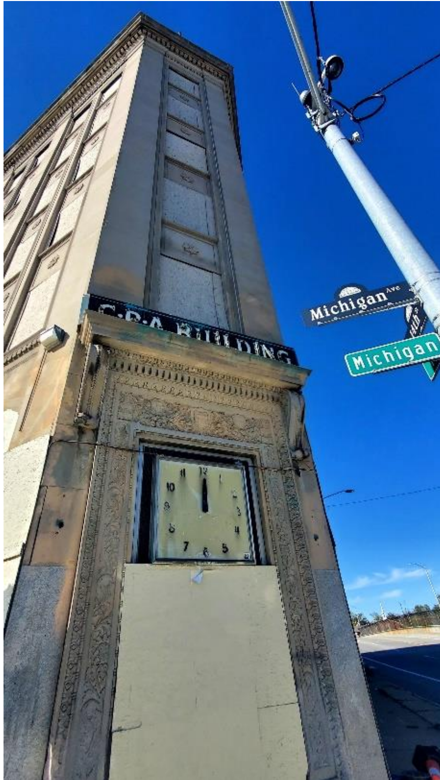
Main entrance at northwest corner of Michigan Ave. and 14th St., looking north (November 2024).
