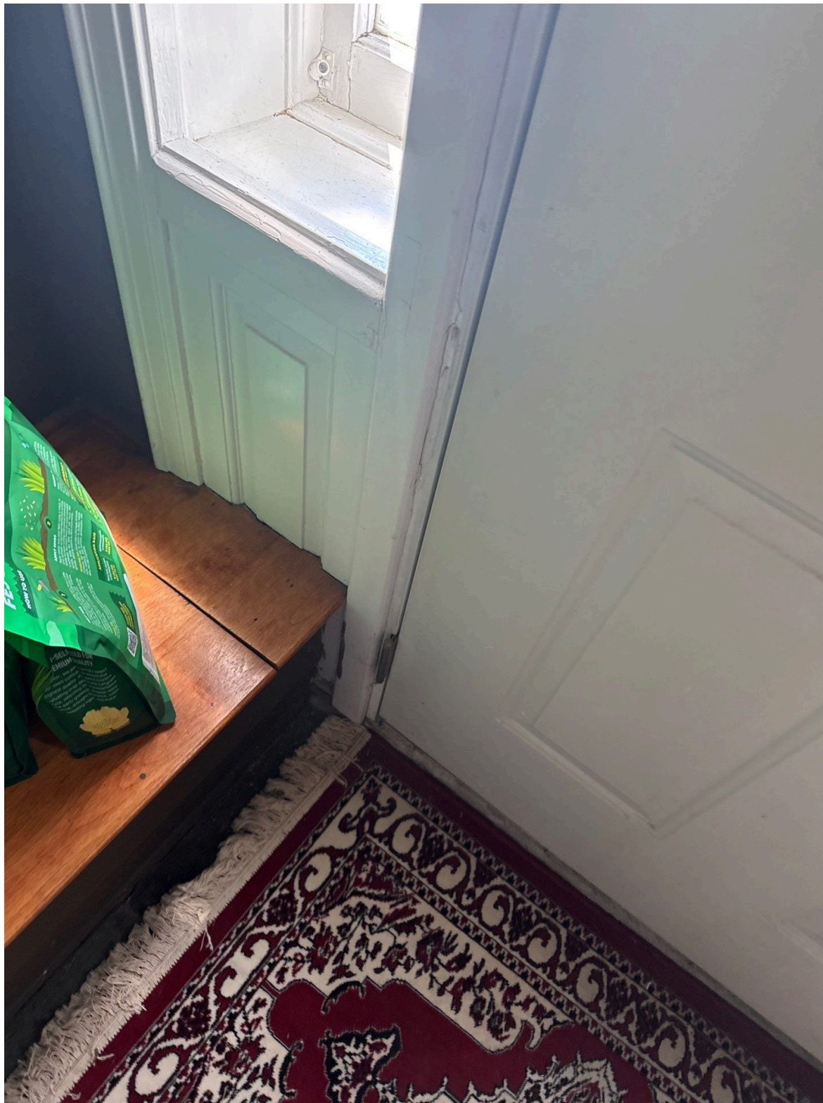
John Lacroix: Entry Doors 15014 Piedmont St • Detroit, Michigan 48223
