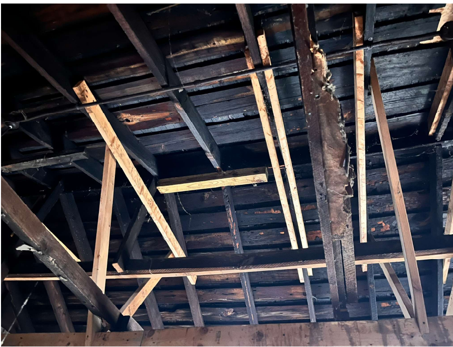
IMAGE 18: TEMPORARY SISTER SUPPORTS FOR EXISTING RAFTERS - UNKNOWN WOOD CONDITION DUE TO LONGTERM WEATHER EXPOSURE
