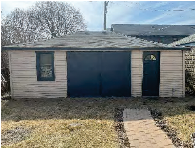
Existing photo - north, rear yard side
