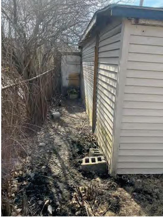
Existing photo – east side
