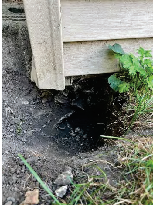
Test pit showing bottom of slab +/- 8"
