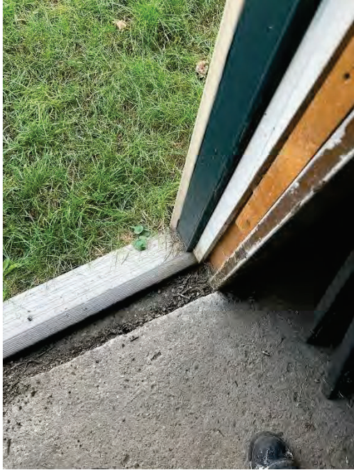
Level of exterior grade compared to slab
