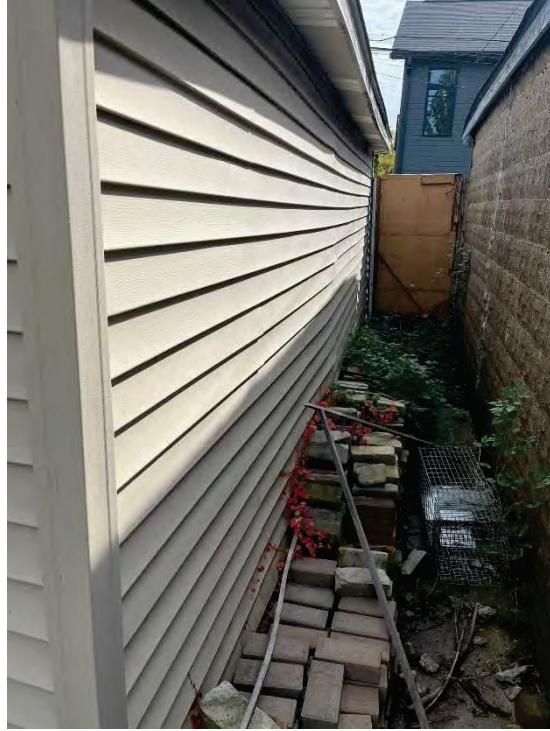
Existing photo – west side
