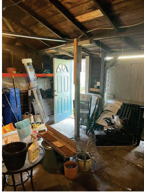
Excessive deflection in supporting member
