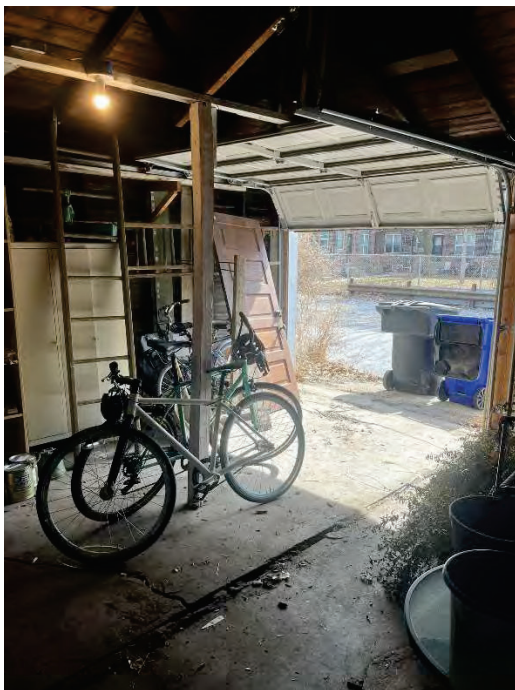
Temporary column installed to support roof
