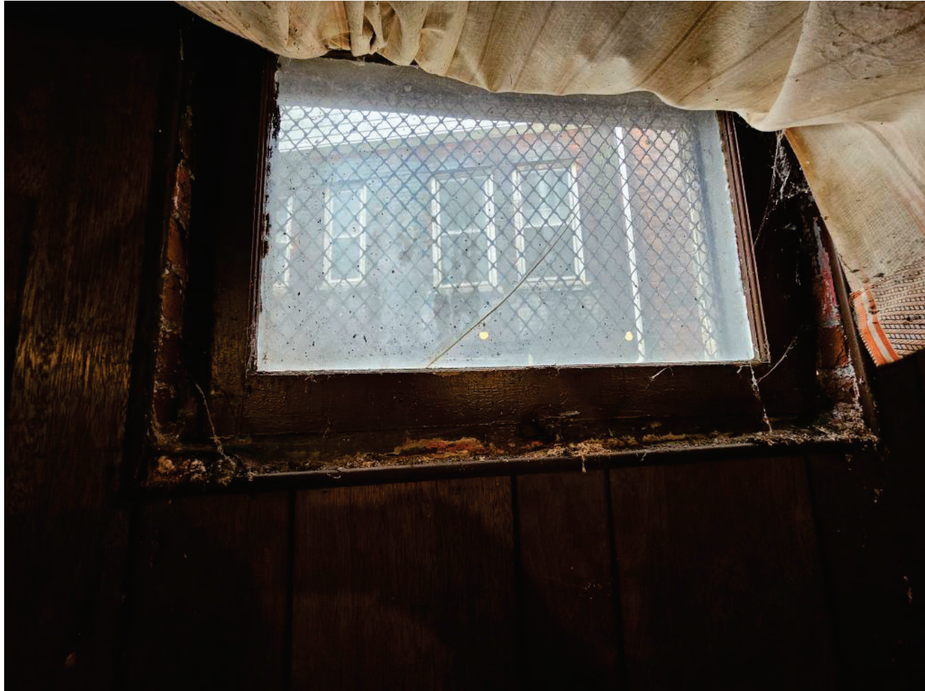
Unit 103 (basement) Exterior / Interior
