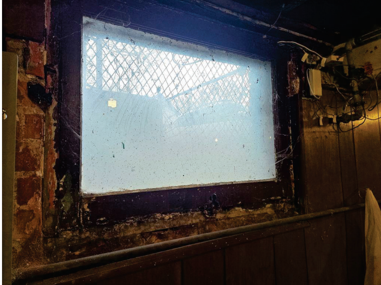
Unit 104 (basement) Exterior / Interior
