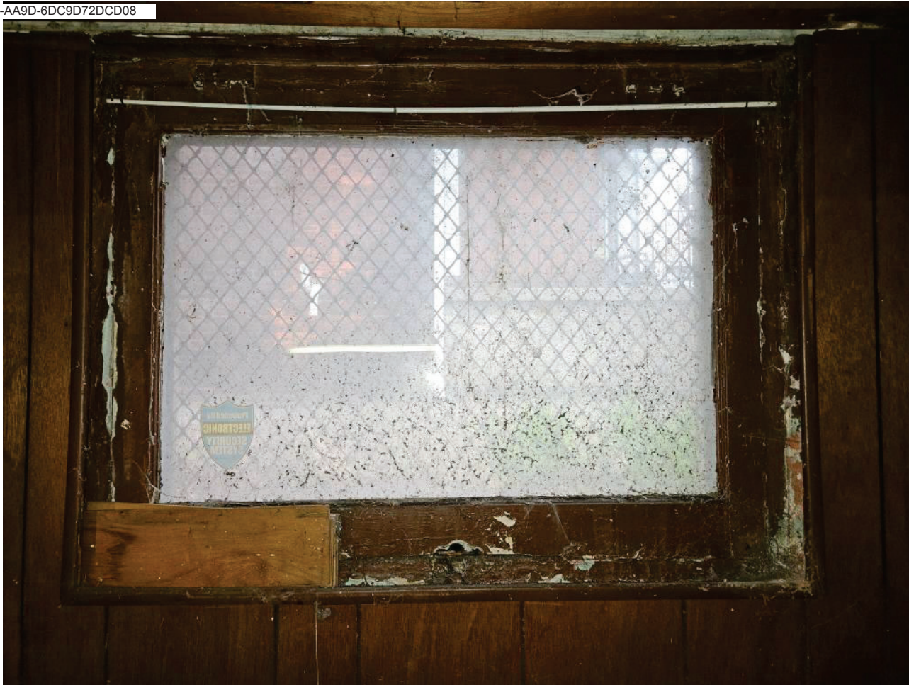
Unit 100 (basement) Interior
