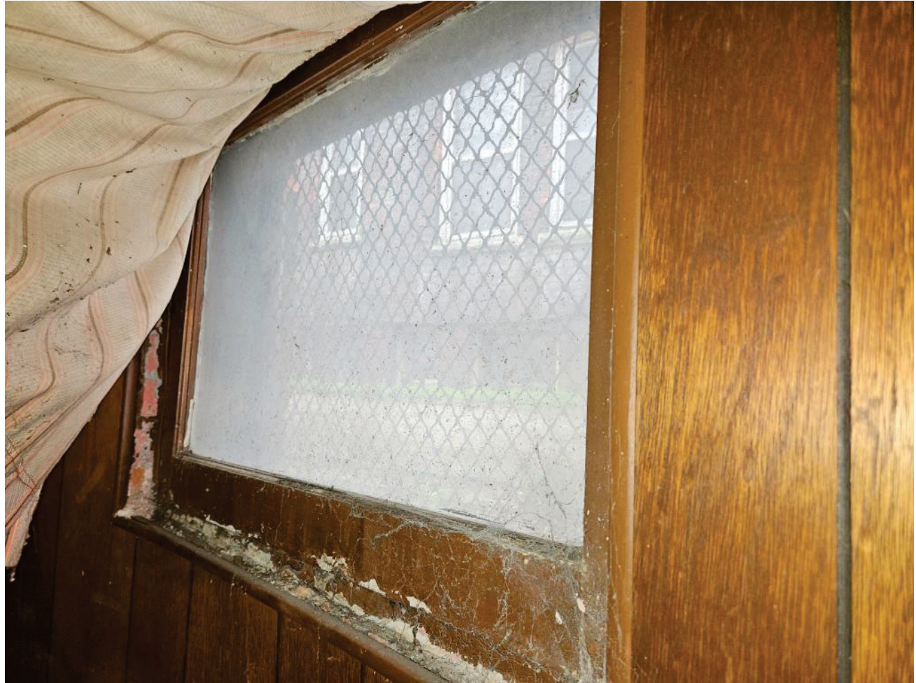
Unit 102 (basement) Exterior / Interior
