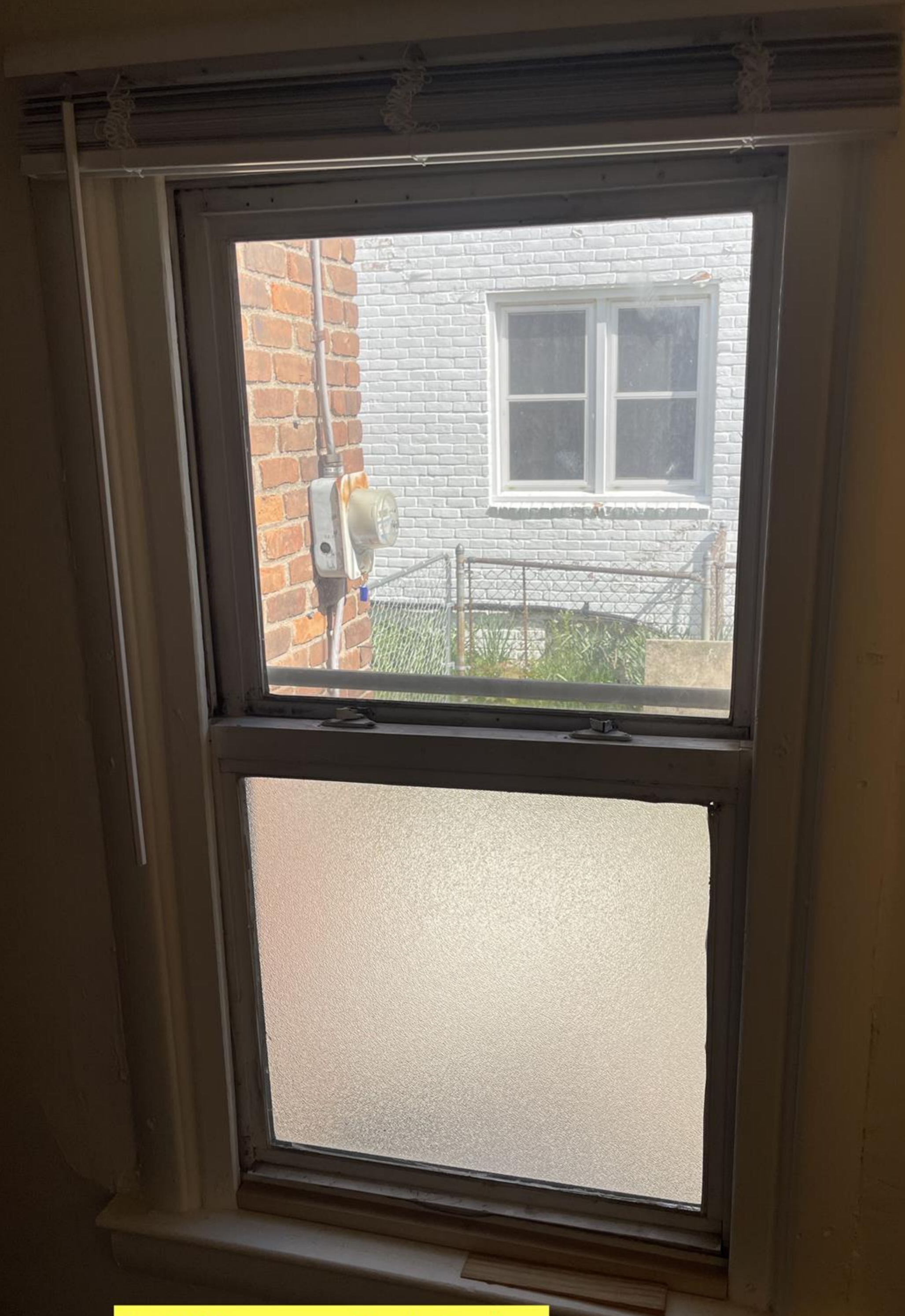
Addition north interior
