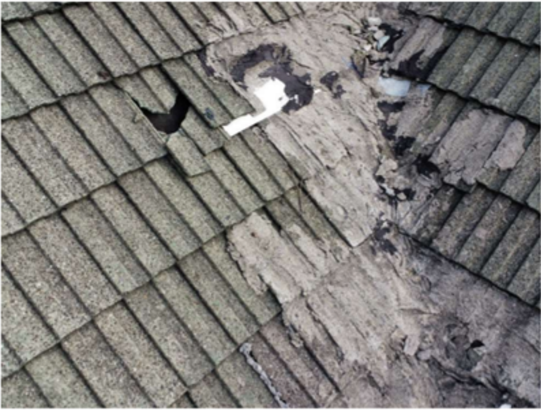
Photograph 11: View of historical repairs.
