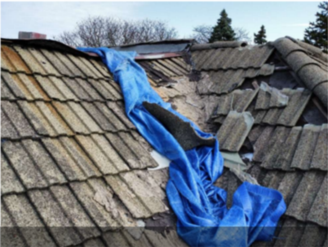
Photograph 15: View of displaced roof tiles on roof slope C.
