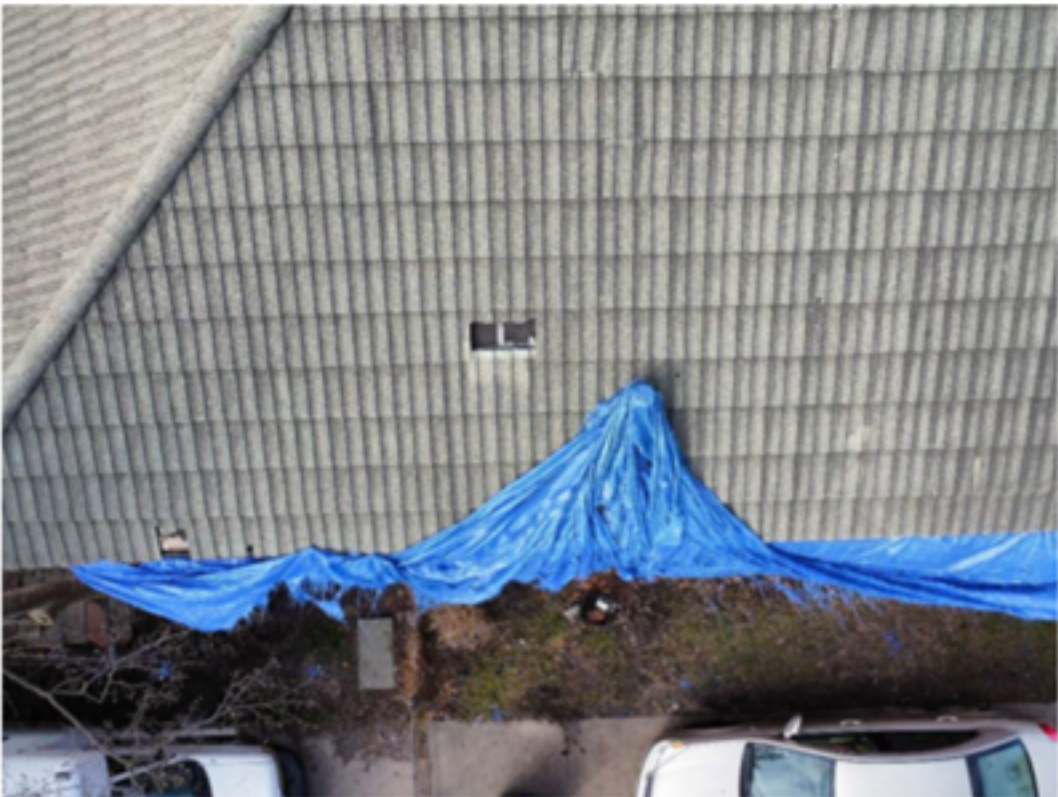
Photograph 13: View of missing tiles on roof slope R.
