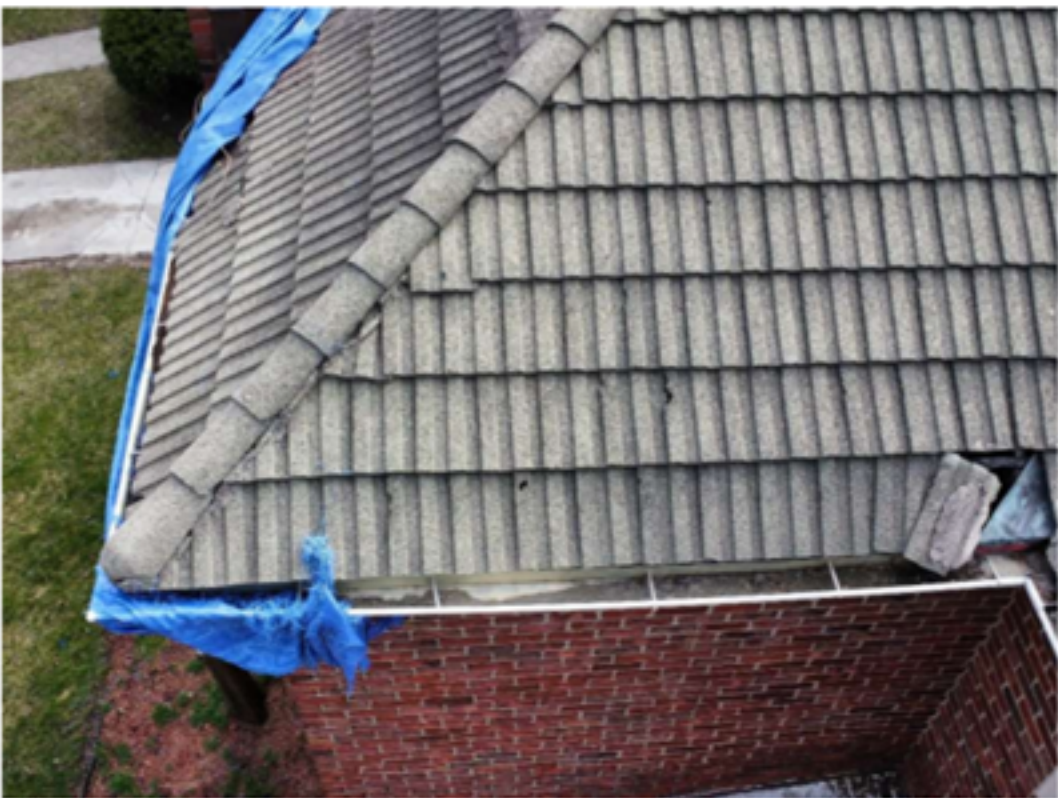
Photograph 16: View of sliding tile on roof slope N.
